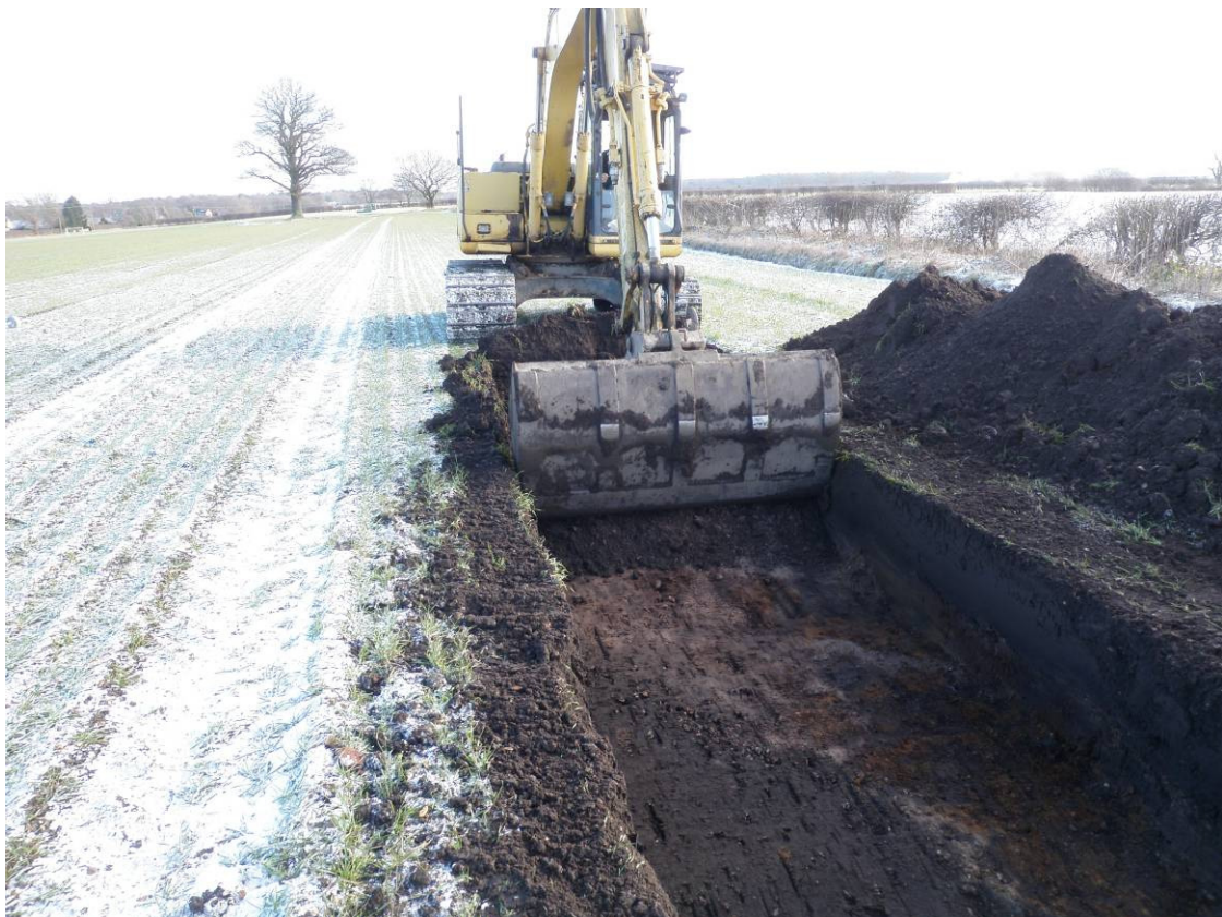
Plate 2 – Working shot of Trench 6, looking northeast
