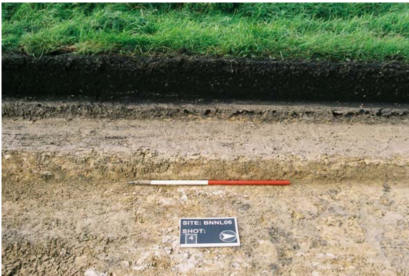
Plate 5 - Section through planed road surface, looking west
