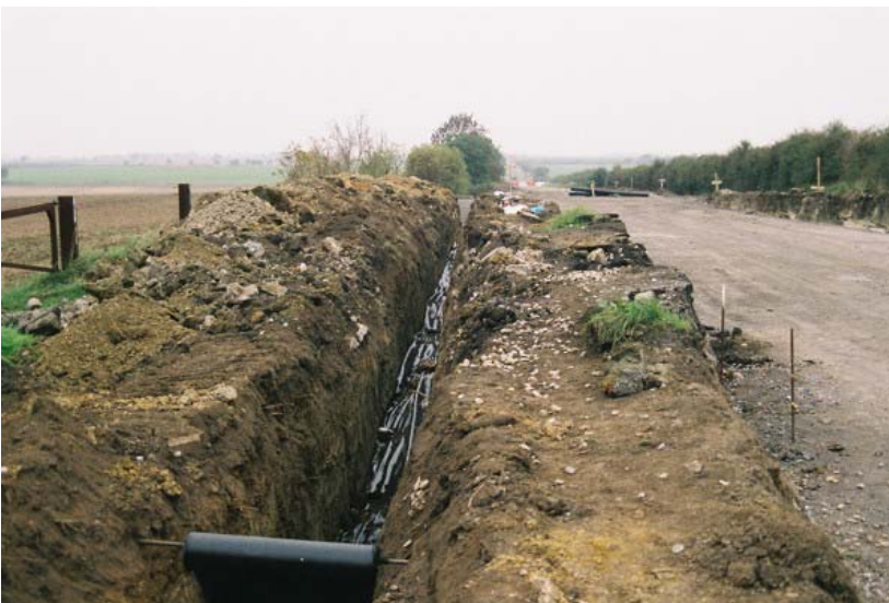
Plate 3 - General view of drainage channels, looking north
