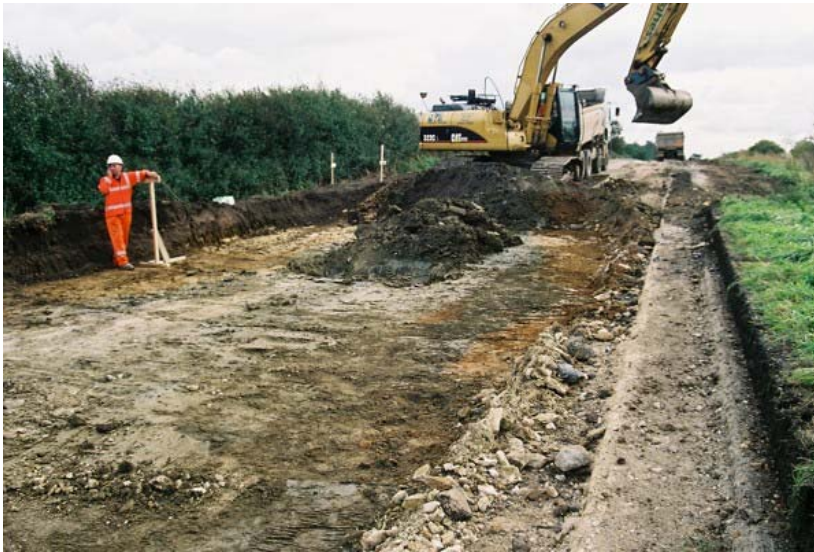
Plate 6 - Stripped area showing linear [1015], looking south
