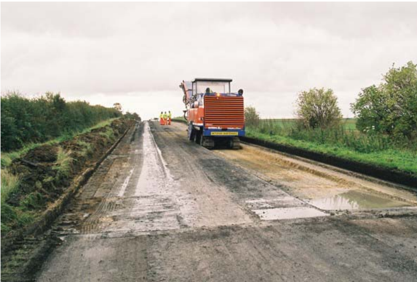
Plate 2 - General view of road planing, looking south
