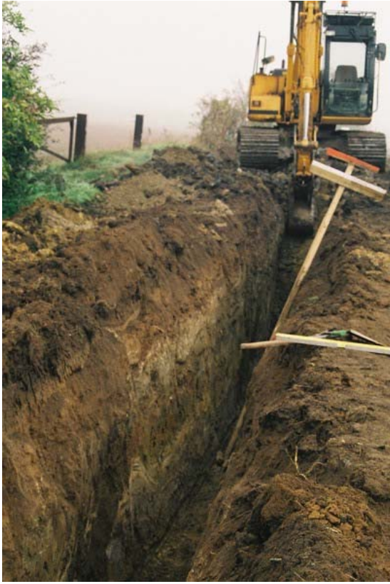
Plate 4 - Excavation of drainage channels, looking north
