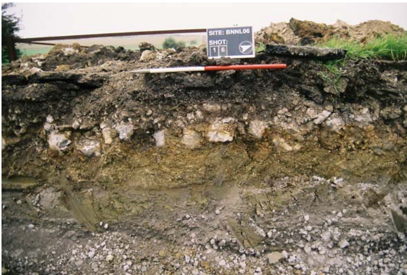
Plate 11 - Section 2, looking west
