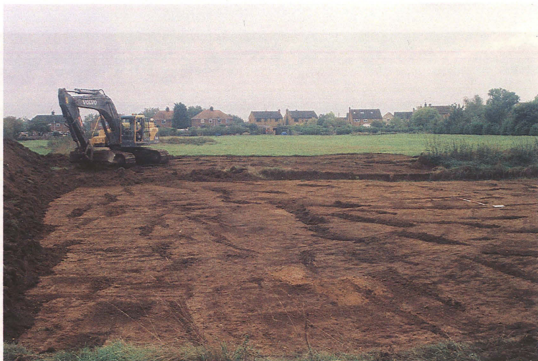
Plate 1 General shot of stripping in progress
