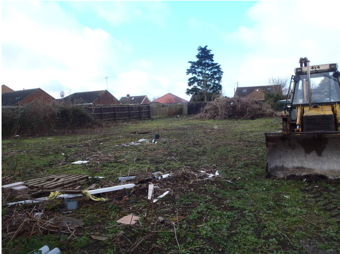
Plate 1 – General view of site looking southeast
