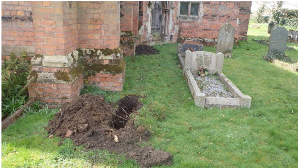
Plate 5. North of the church, looking west.
