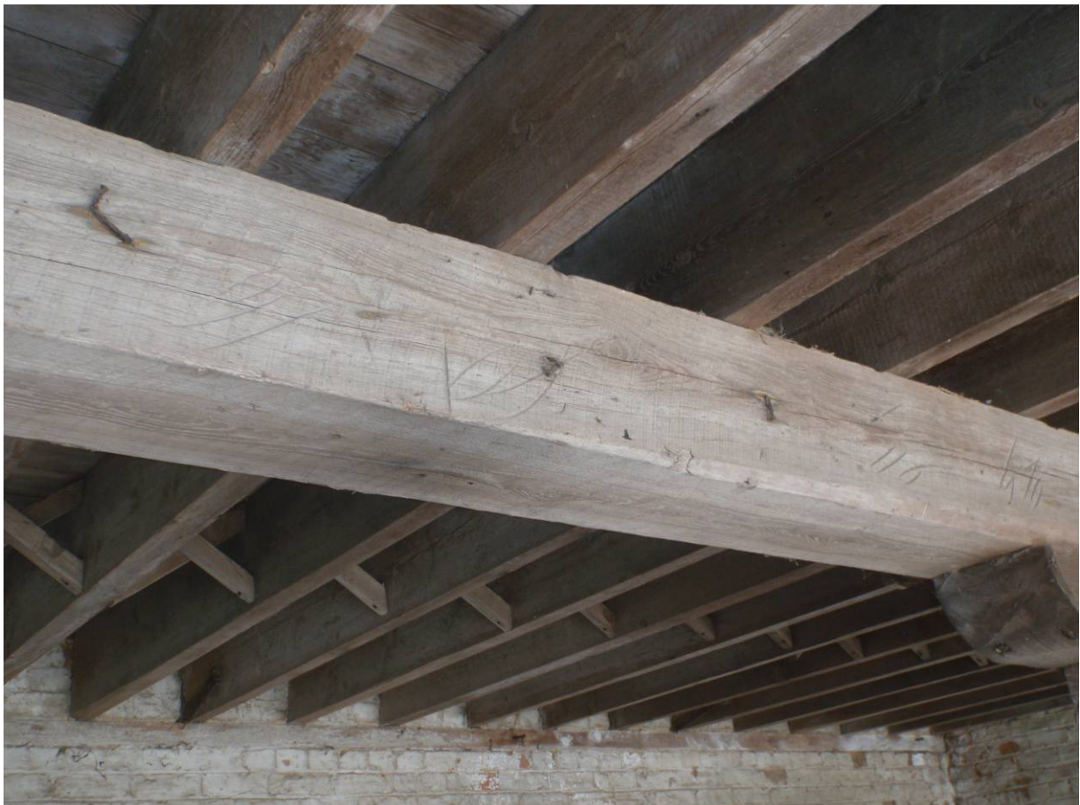
Plate 13 Possible 'Baltic' importers' marks on beam, looking northwest
