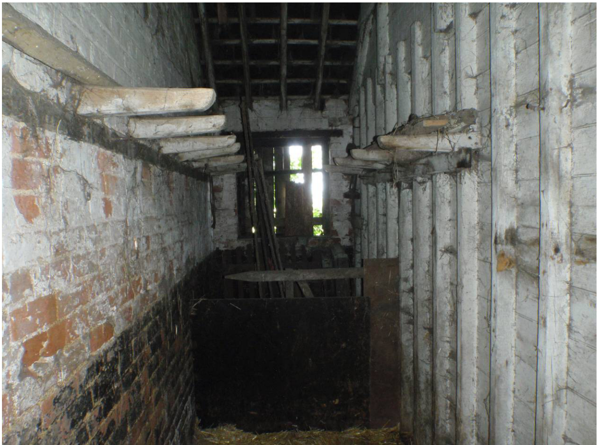
Plate 21. North range, Room 3, looking north
