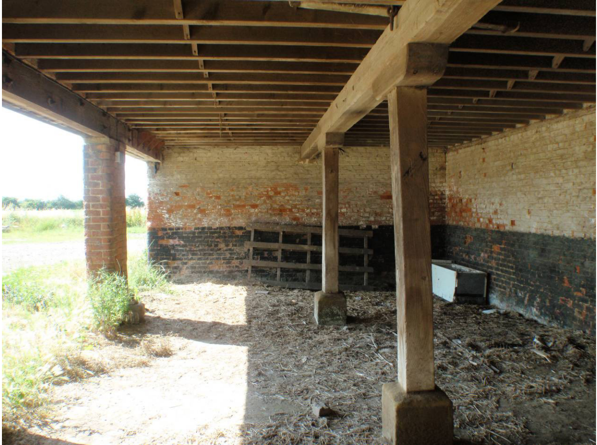
Plate 10. Interior of northern compartment of east range, looking south
