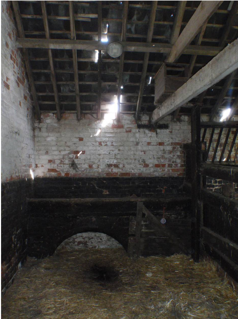
Plate 19. North range, western compartment (Room 1), looking north
