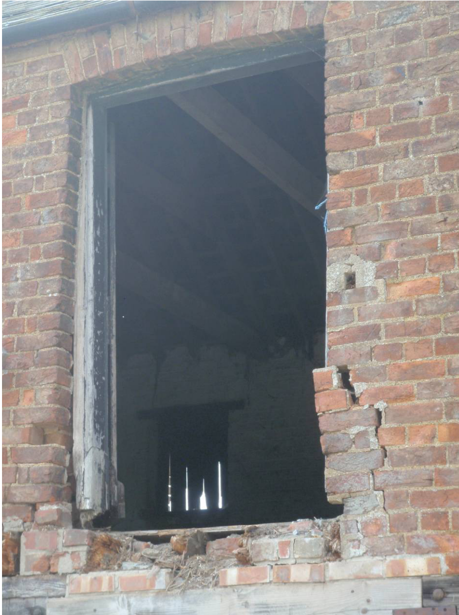
Plate 14. View into upper storey, east range, looking southwest
