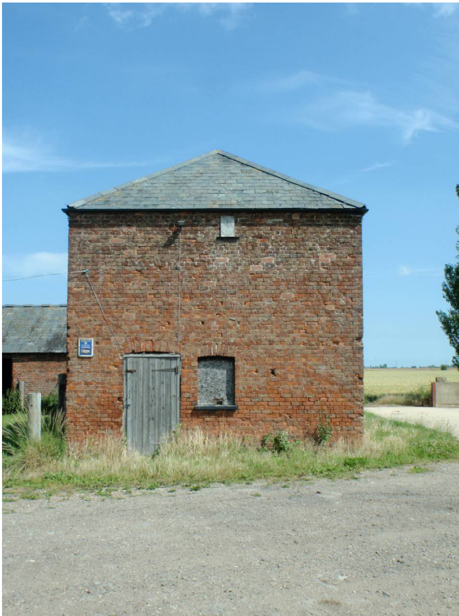
Plate 5. Eastern range, southern elevation, looking north
