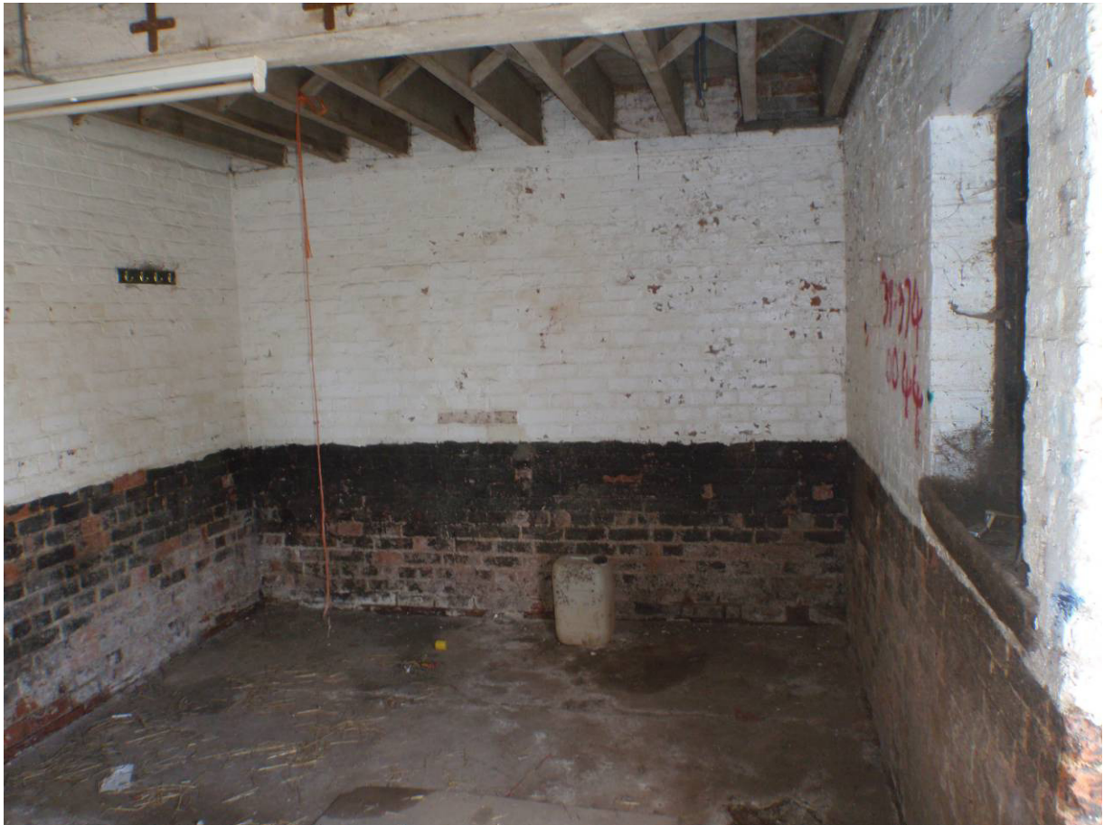
Plate 8. Interior of southern room, east range, looking east
