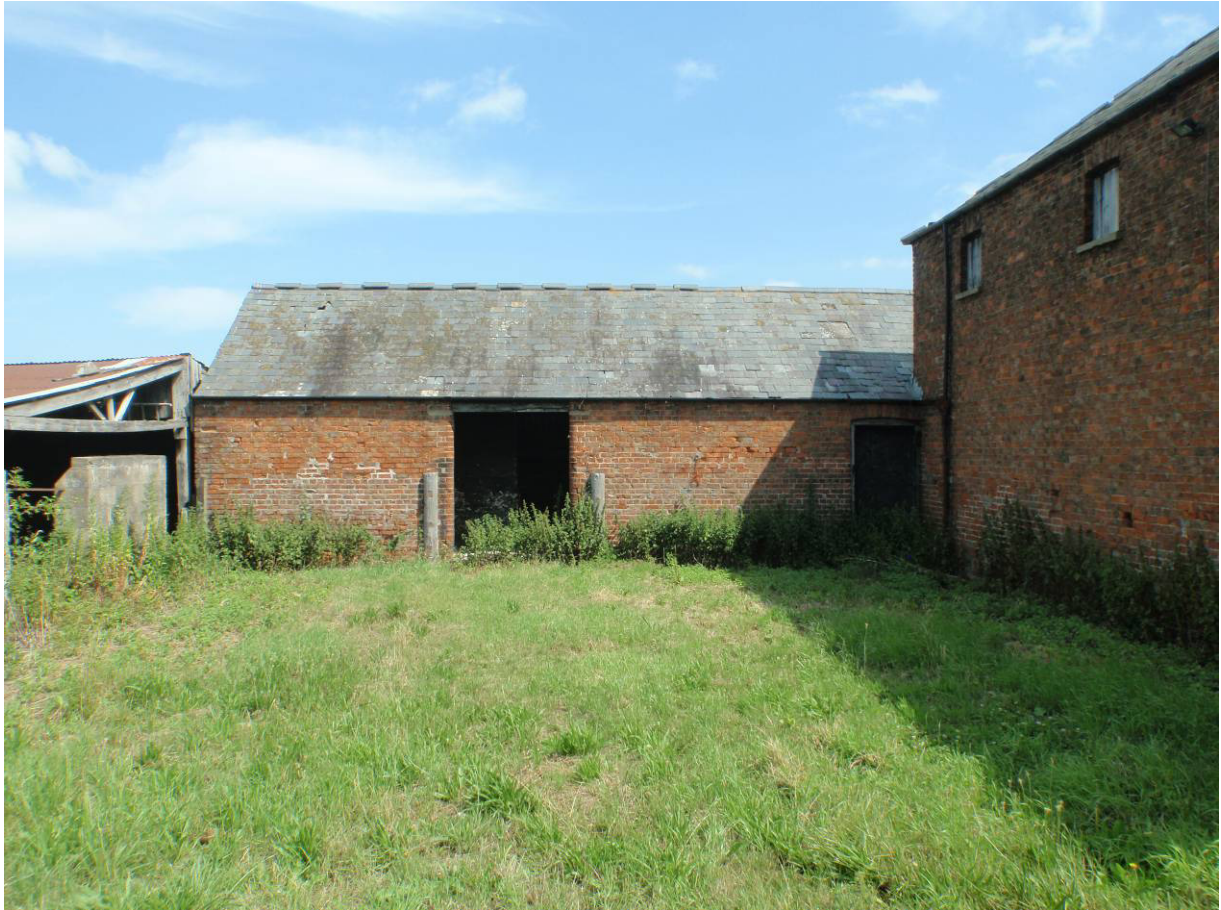
Plate 15. Northern range, south elevation, looking north
