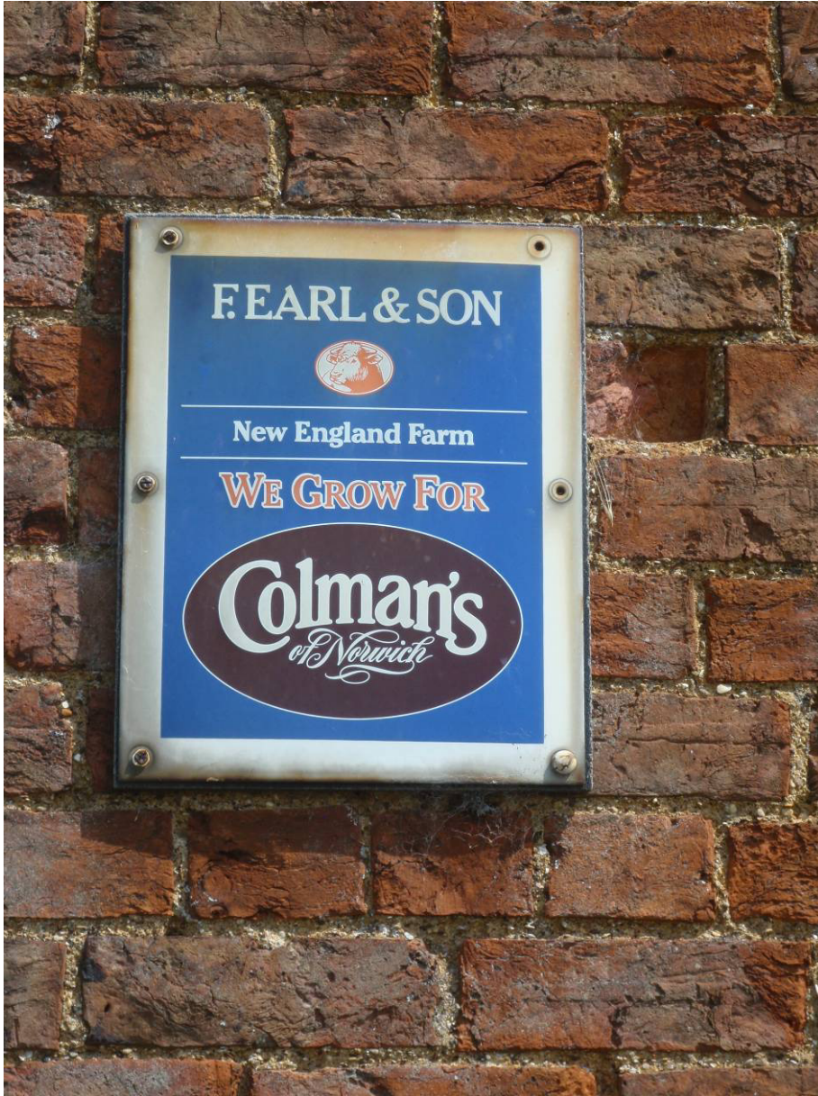
Plate 6. Detail of advertising panel on south elevation
