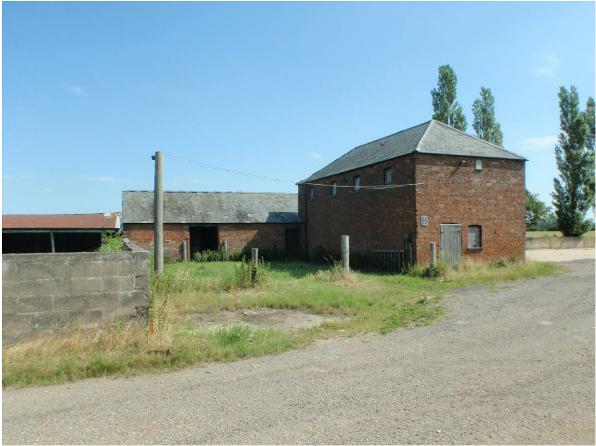
Plate 3. The recorded buildings, looking northeast
