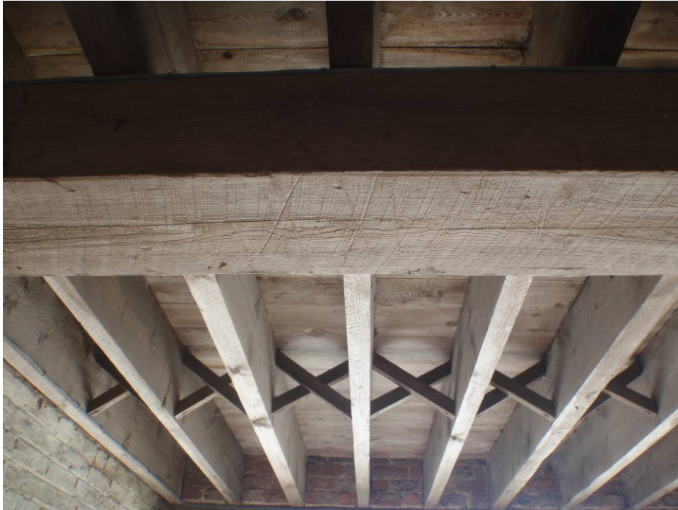
Plate 12. Underside of beam showing incised Roman numerals, looking east
