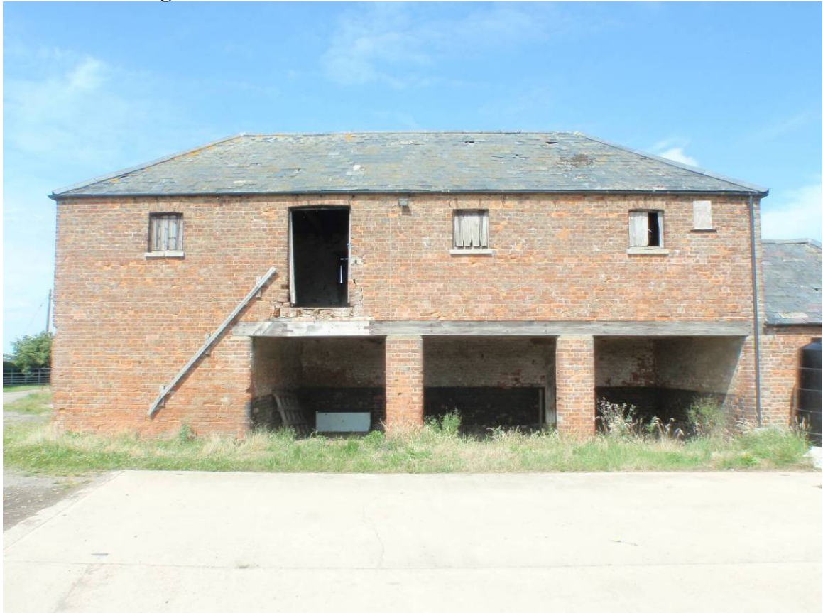
Plate 4. East range, eastern elevation, looking west
