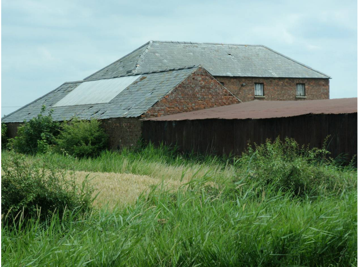
Plate 16. North range, west and north elevations, looking southeast
