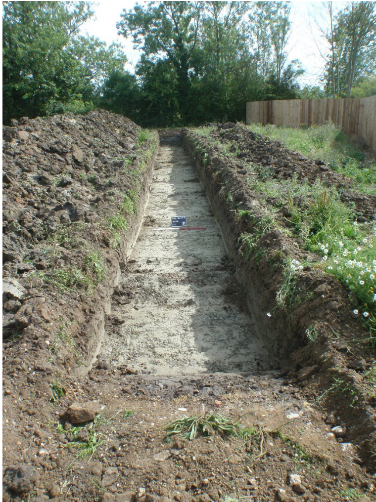
Plate 6 – Trench 4 after excavation, looking south
