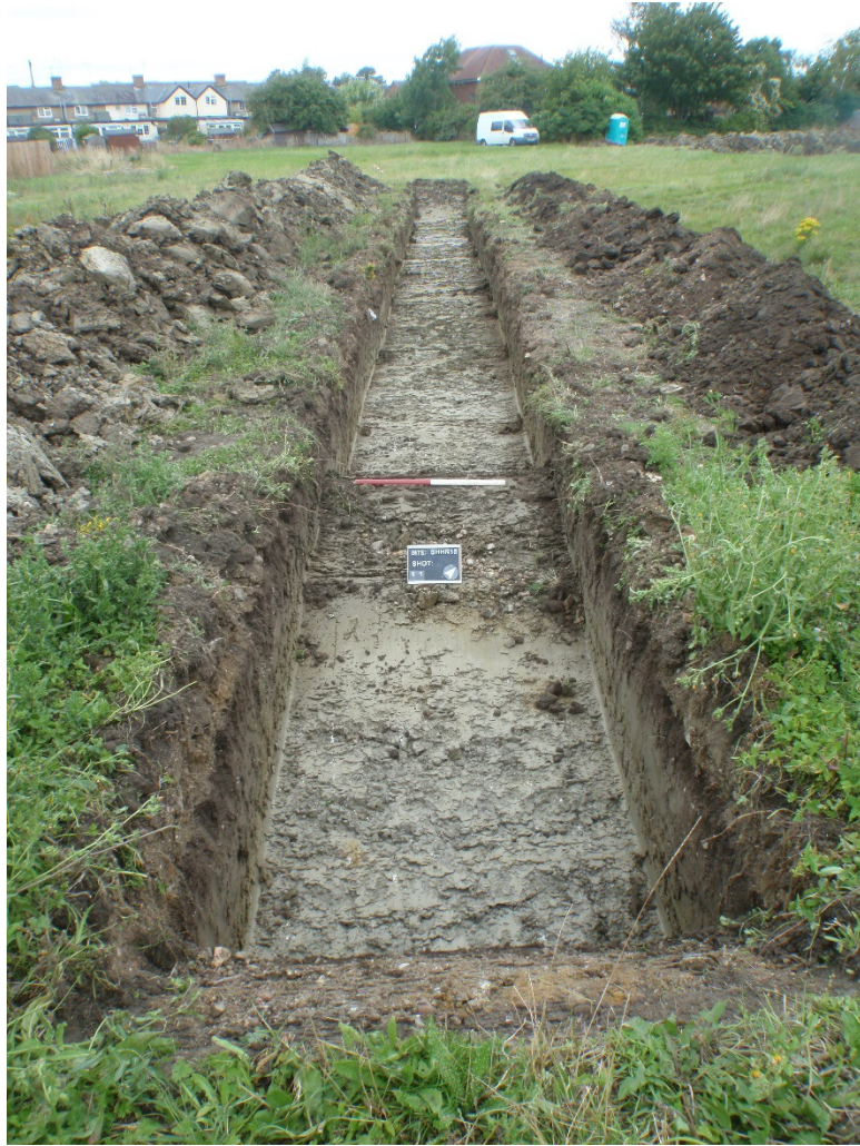
Plate 4 – Trench 3 after excavation, looking northwest
