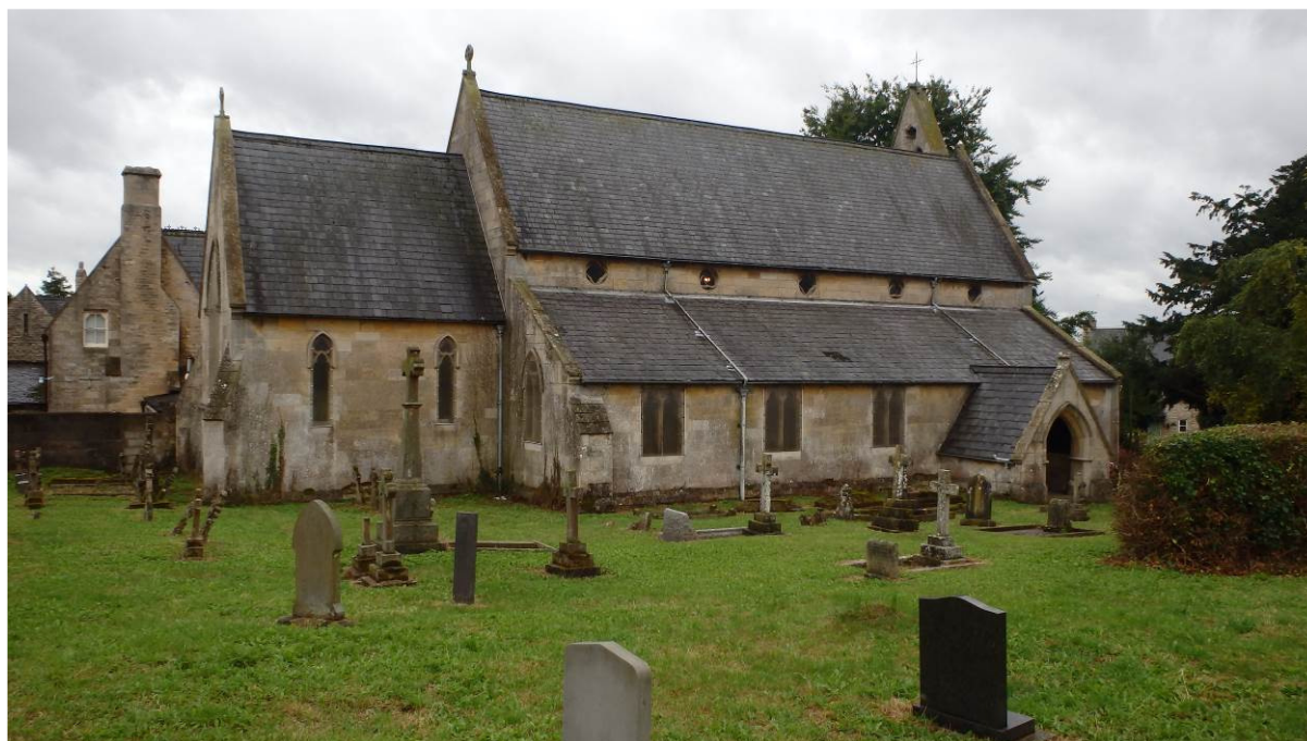
Plate 1. General view of the north elevation of the church.
