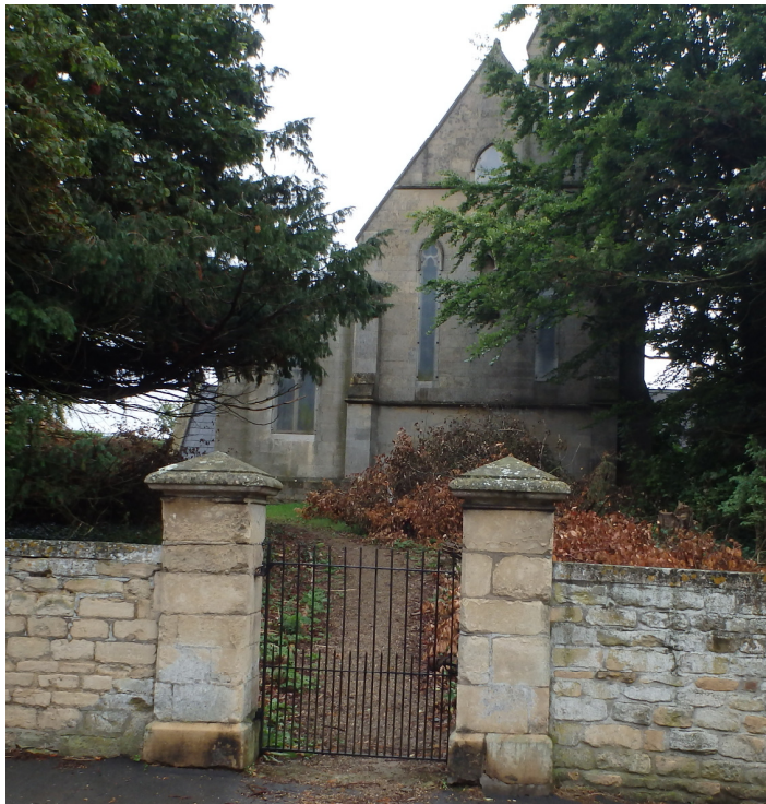
Plate 18. The stone gateposts, to be dismantled and rebuilt further to the north in the western boundary wall
