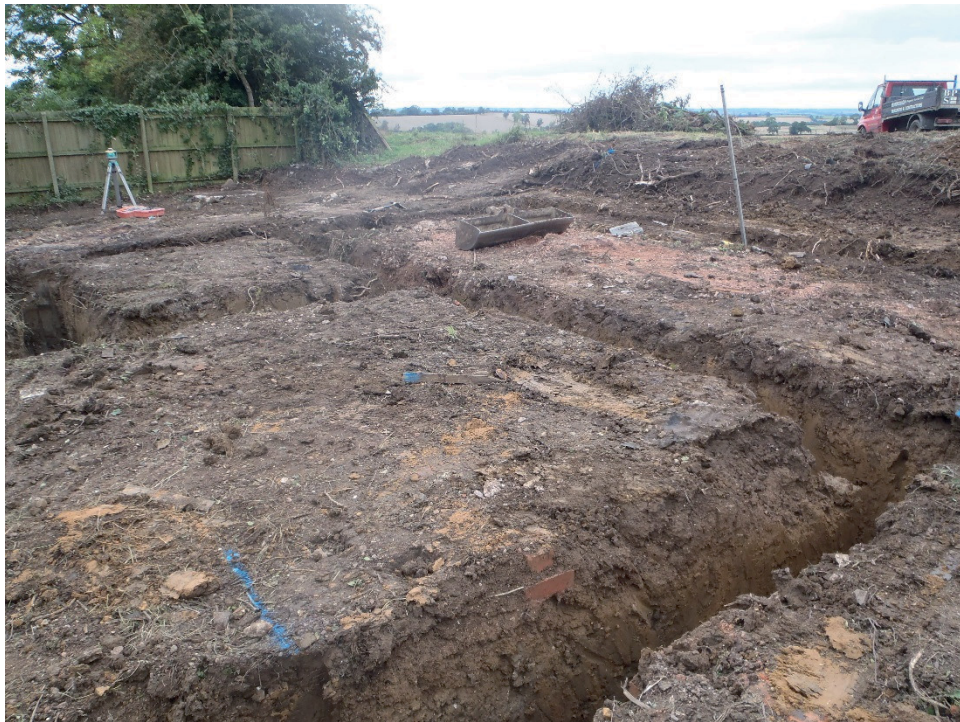
Plate 2 – View across the excavated foundation trenches, looking northwest
