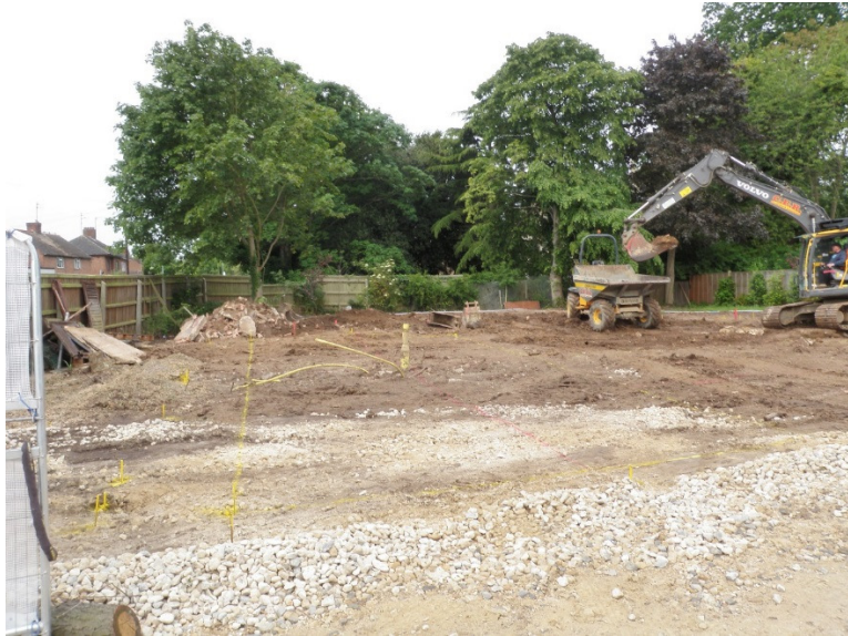
Plate 1. View of house plot at start of excavation looking southwest
