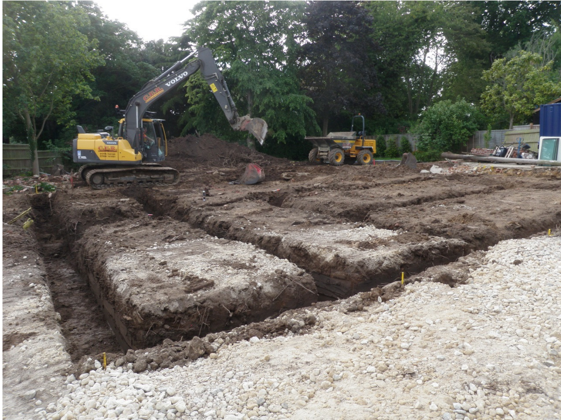
Plate 5. Overall view of house footings looking west
