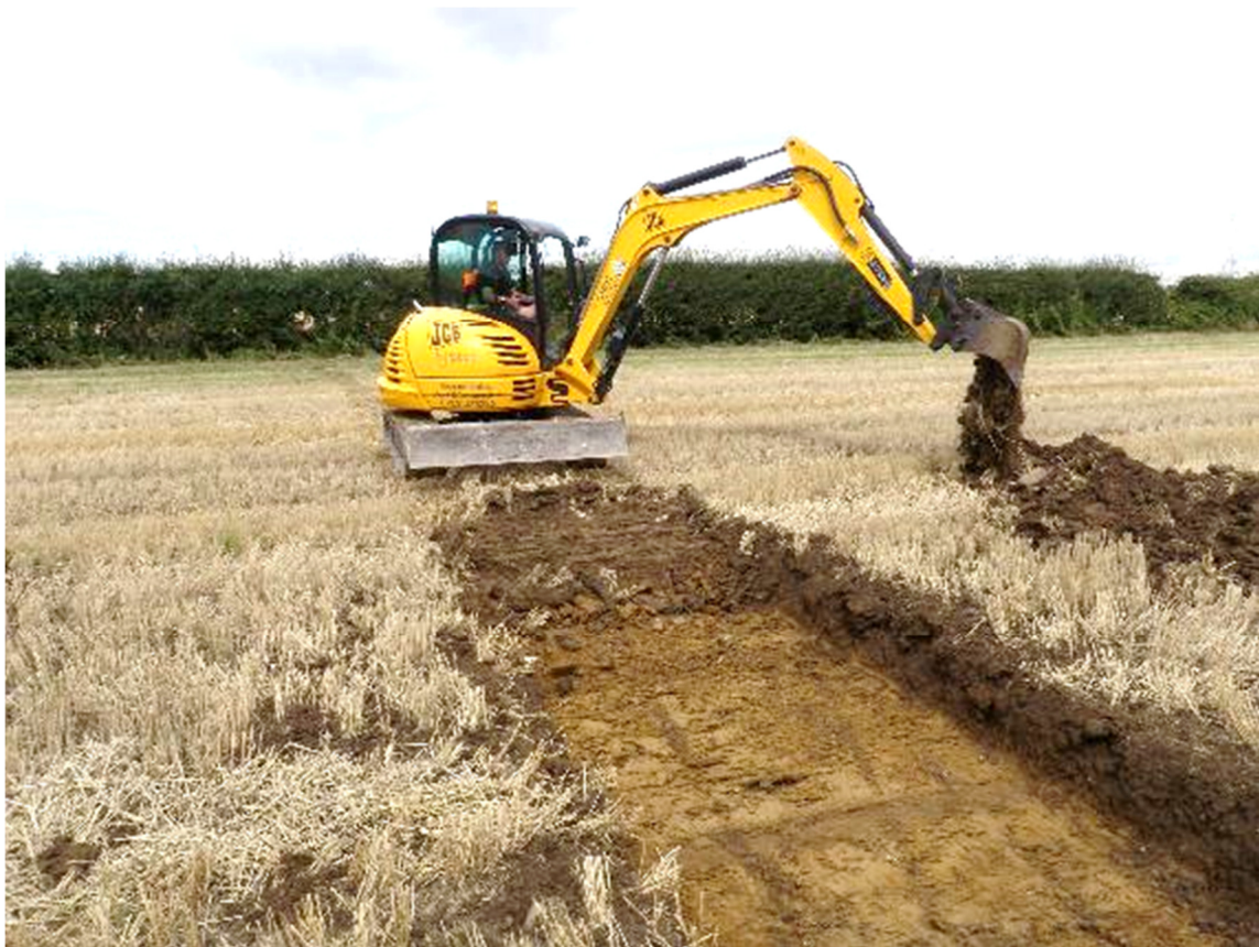
Plate 2. Machining Trench 3 looking north
