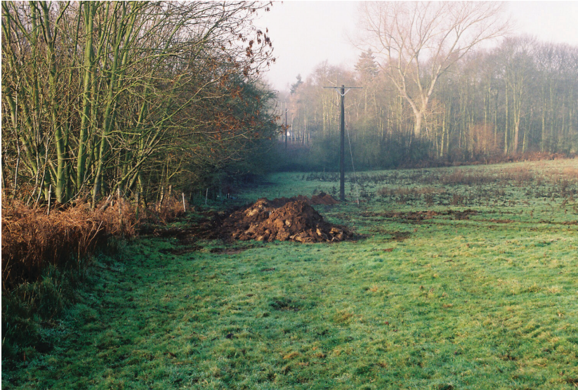
Plate 1 - View showing the extent of the cable trench, looking west
