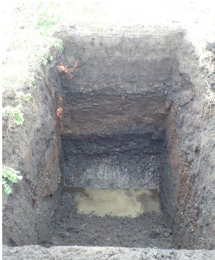
Plate 6 Test Pit 5, looking southeast.
