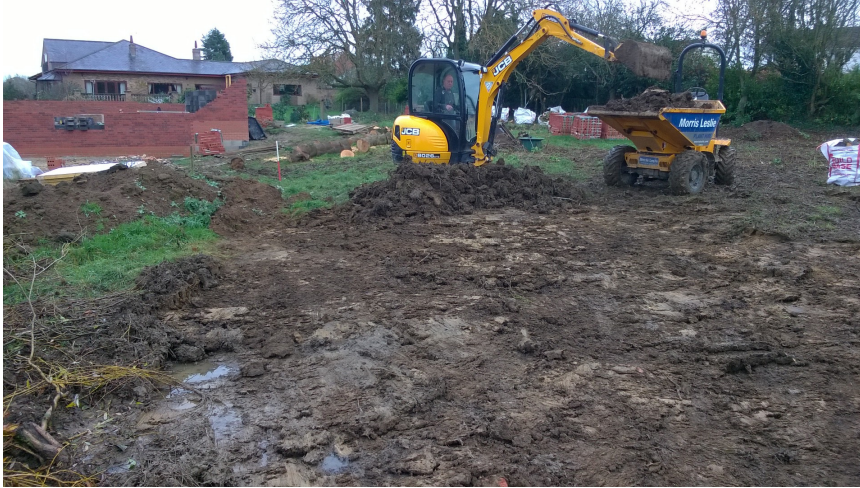
Plate 1. Stripping turf from the house plot looking northeast
