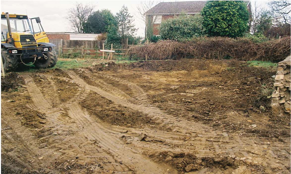
Plate 1 General view of site after levelling, looking north
