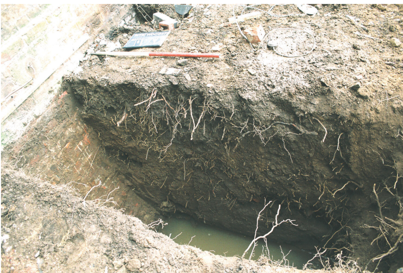
Plate 3 - Section 2 showing the foundations of the church, looking southeast
