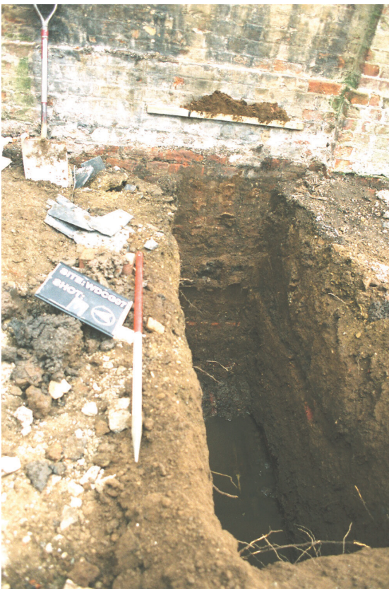
Plate 2 - Section 1 showing the foundations of the church and wooden raft, looking east
