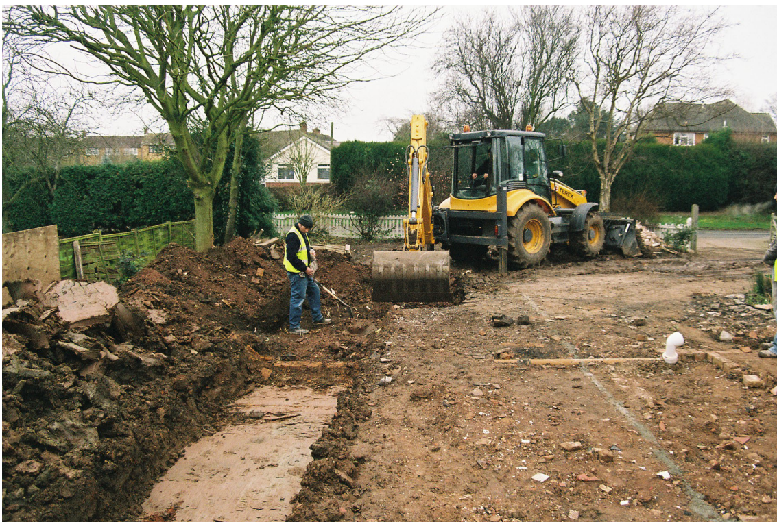
Plate 2: Machining Trench 1 looking NW
