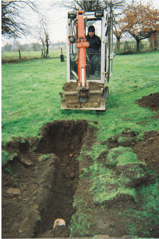
Plate 1 - View of the drainage trench during excavation, looking north
