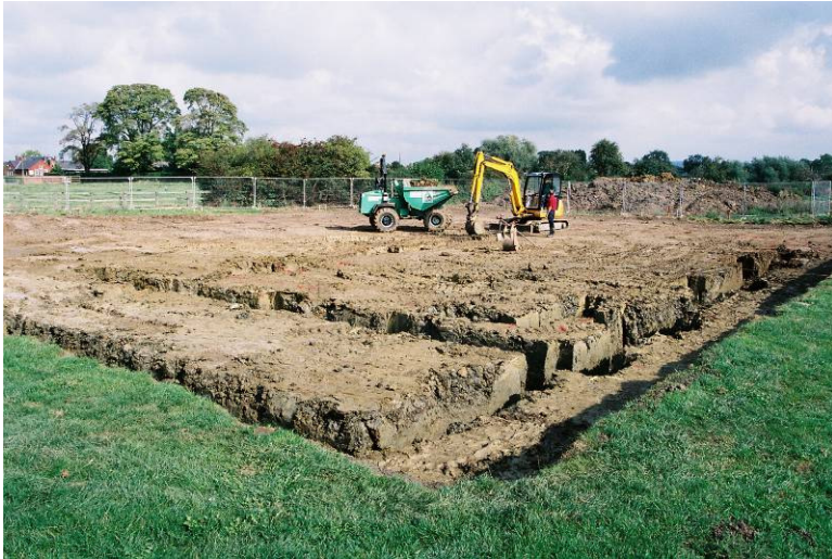
Plate 4 - View showing the excavation of the foundation trenches, looking northeast
