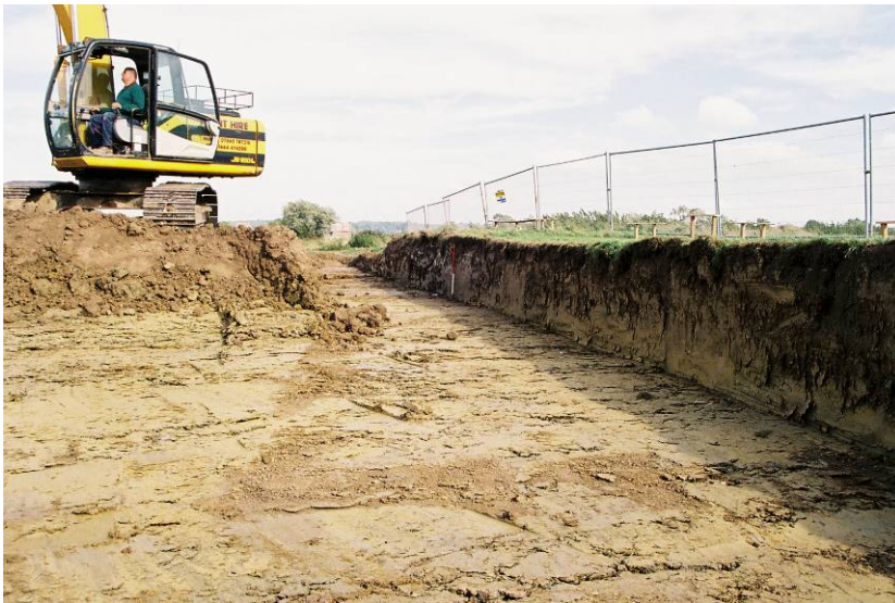
Plate 2 - Section 1 showing the earthwork ridge across the site, looking southeast
