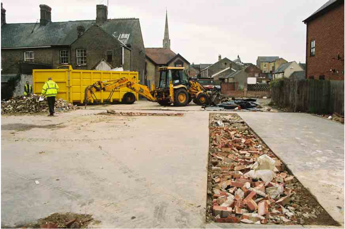
Plate 1 General view of the site showing infilled vehicle inspection pits, looking south
