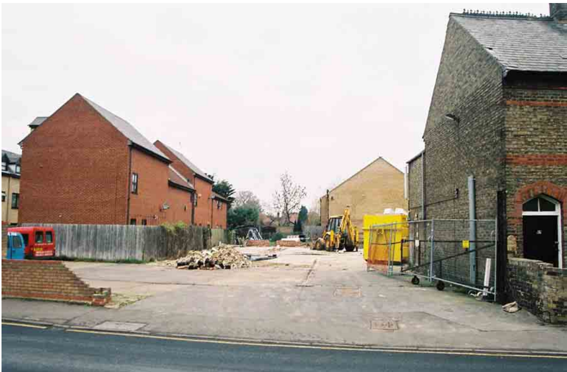
Plate 2 General view of the site from East Street, looking North
