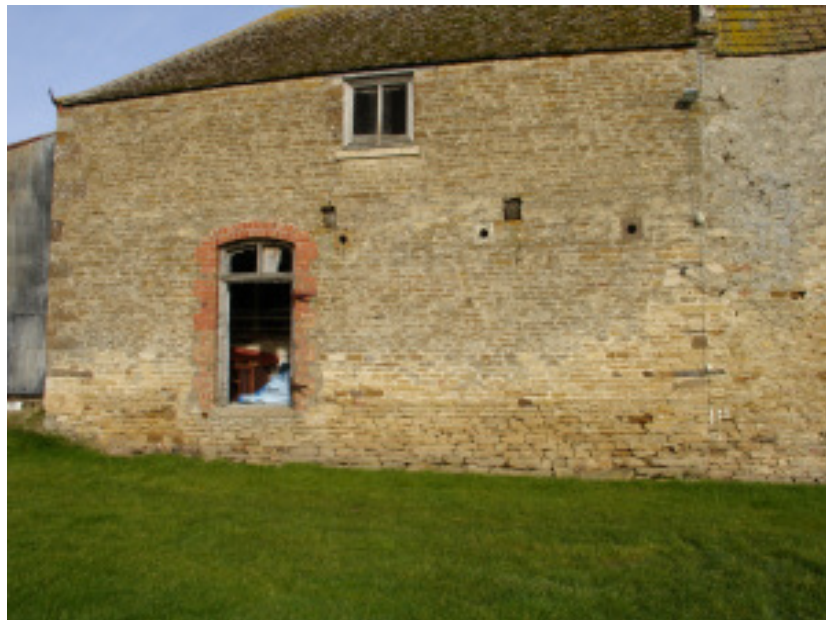
Plate 10 - South elevation of the barn showing inserted doorway, looking north
