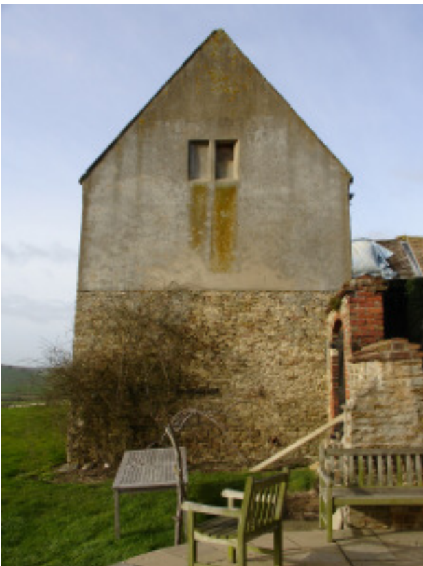
Plate 3 - East facing elevation of the dovecote showing blocked windows and rendering, looking west
