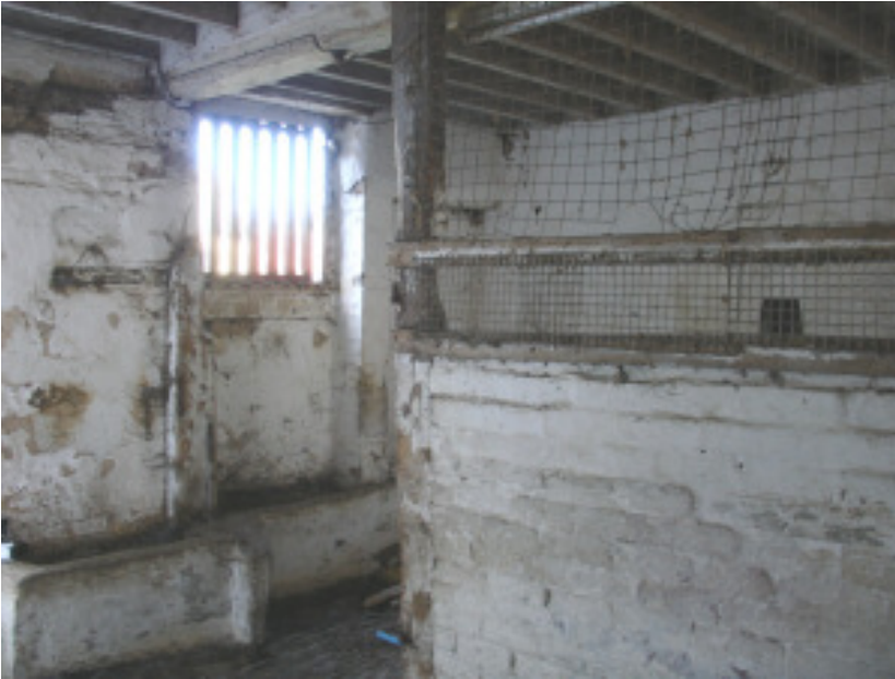
Plate 10 - Interior view of the east room of the barn showing brick partition and stone feeding troughs, looking northeast
