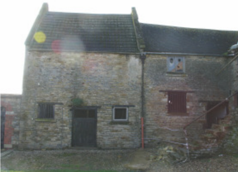
Plate 2 - North facing elevation of the dovecote showing gable arrangement and inserted doors and windows, looking south
