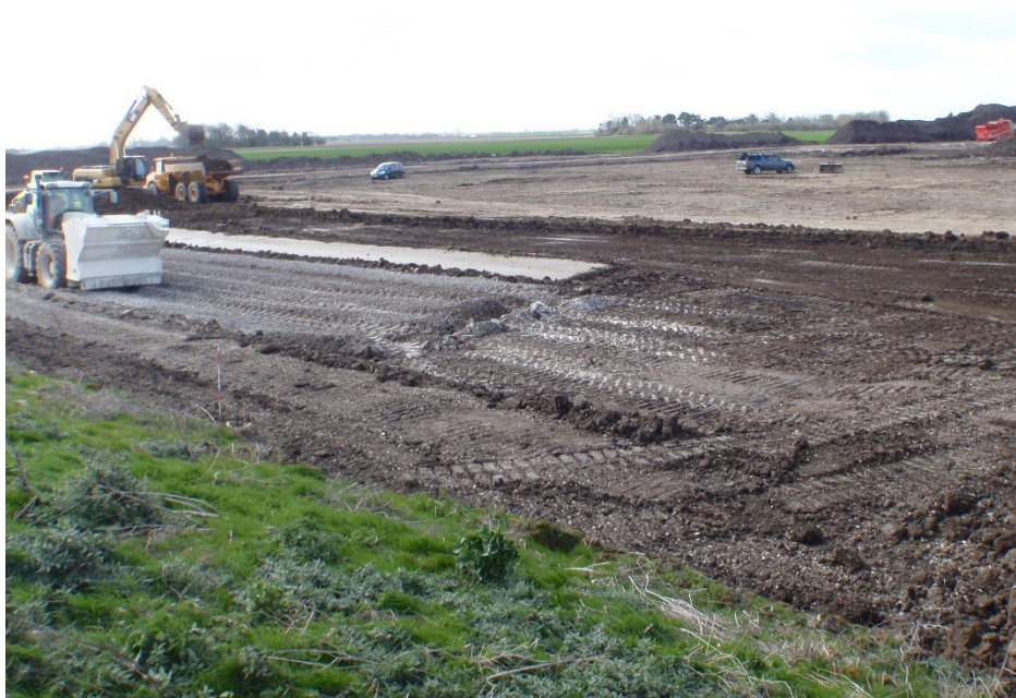
Plate 1: Working shot of site, looking southwest
