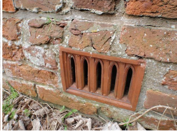
Plate 8 Detail of the ceramic vent at the base of the extension to the North-South Range
