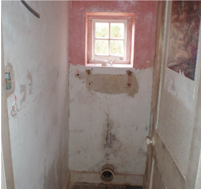
Plate 34. Room 6, used as a lavatory and the probable recycled window within a mid-20 th century aperture
