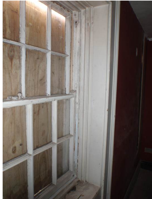
Plate 17 (above). Detail of the Victorian sash window within the Georgian Frame. The runners for the previous sash cords are visible just inset from the present window
