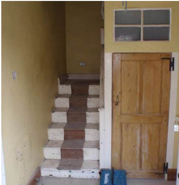
Plate 19 General view of the vestibule/hallway
