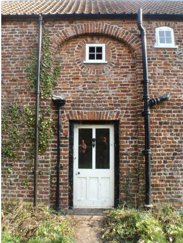
Plate 2 (left). Detail of the central doorway within the two storey recess under the three centre arch. The bulls-eye opening has been partly infilled and a small square window inserted
