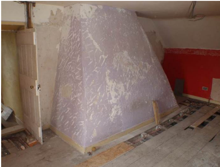
Plate 38. The large, cambered chimney breast in Room 8 above the inglenook fireplace on the floor below
