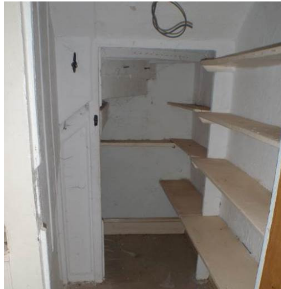
Plate 20 The under-stairs cupboard with the fitted shelves
