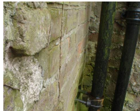
Plate 13 (below). Detail of a protruding brick, cut off within the oven feature
