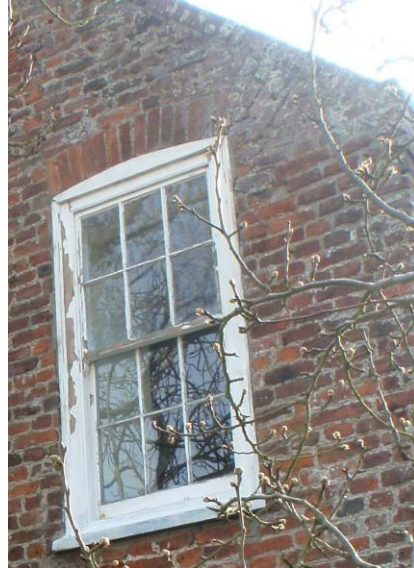
Plate 15 (below). Detail of the upper window cutting the triangular section showing that it is a later insert
