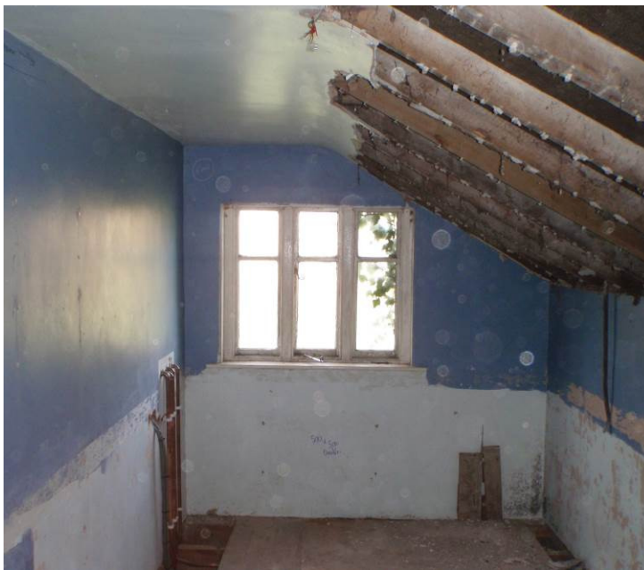
Plate 43. Room 10, showing the exposed rafters and the three light window on the west wall
