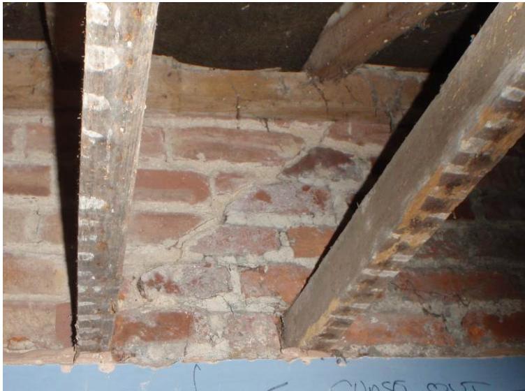
Plate 44. Internal view of the north gable end of the upper part of the North-South Range showing the eaves line of a previous northern extension
