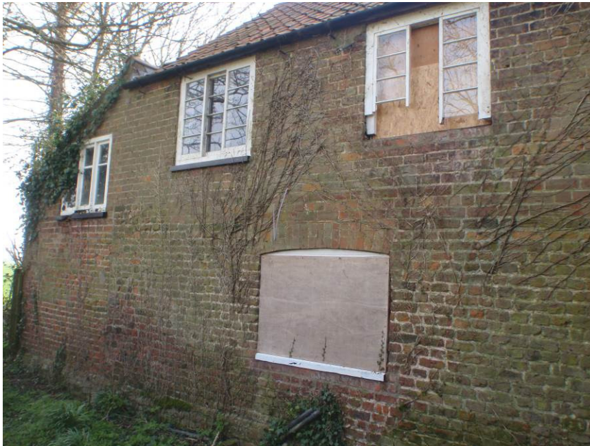
Plate 11. General view of the west elevation of the North-South Range
