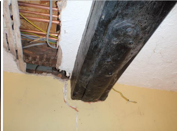
Plate 26. A substantial iron tie on the ceiling beam in Room 3
