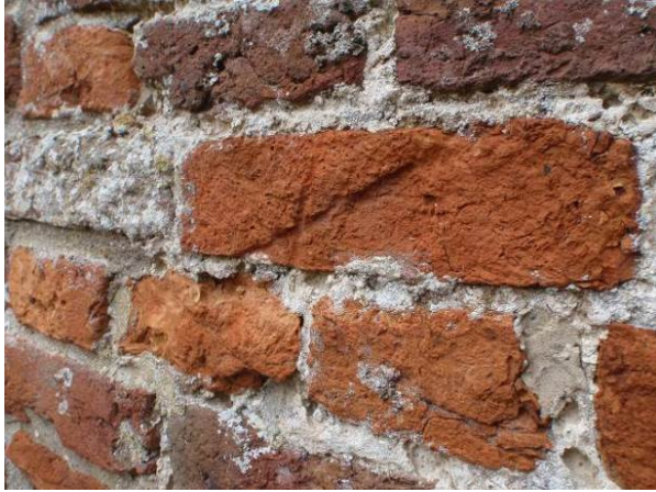
Plate 7 Detail of the 19 th century brick in the northern extension to the North-South Range showing the diagonal stack marks
