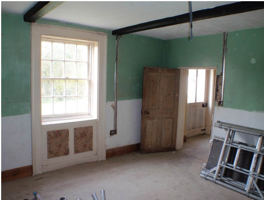
Plate 21. General view of Room 2 looking toward the vestibule/hall and showing the eight over eight Victorian sash window in the Georgian window surround, and the ceiling beams
