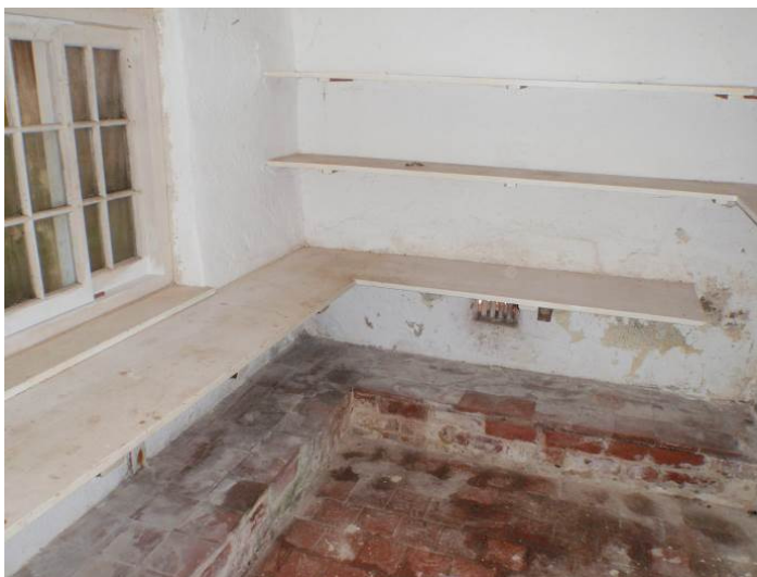
Plate 29. Eastern room of the pantry area with the brick and tile 'cool shelf'. The window on the north wall is a later insert
