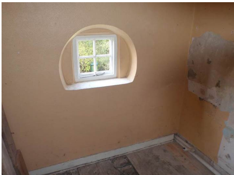
Plate 33. The partly infilled bulls-eye window in Room 5
