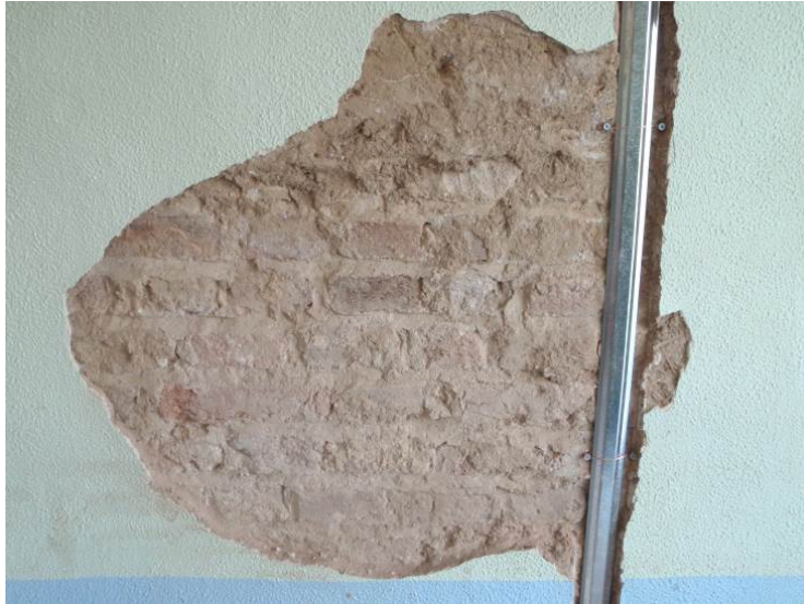
Plate 32. An area of exposed original mud plaster in the south wall of Room 4
