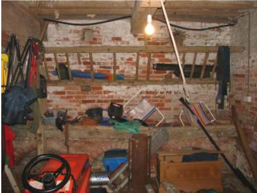
Plate 10 - Eastern stable bay showing manger and hay rack
