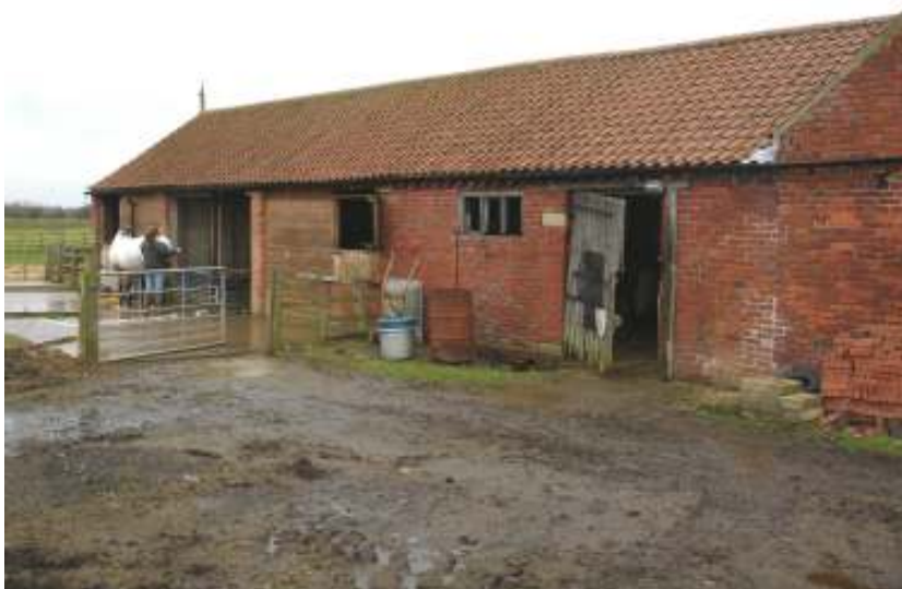
Plate 18 - East facing elevation of the east range with former cart shed to the left
