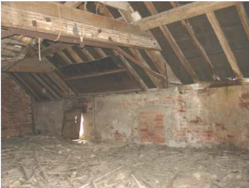
Plate 15 - The granary interior showing the blocked window openings
