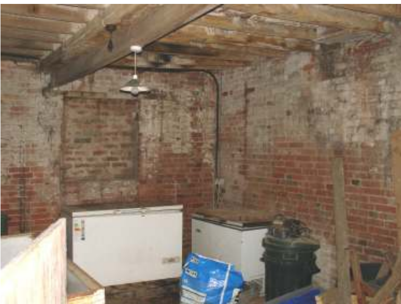
Plate 9 - Interior view of the western ground floor room with blocked doorway
