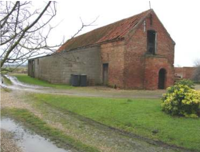
Plate 7 - View showing the concrete lean to on the north side of the north range
