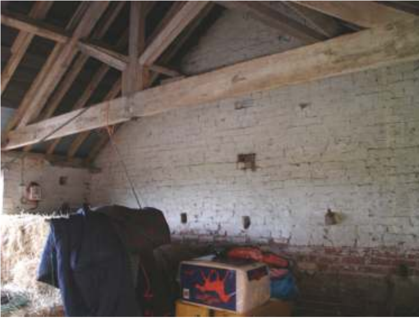
Plate 19 - Interior view of the north room of the east range showing the King post truss roof
