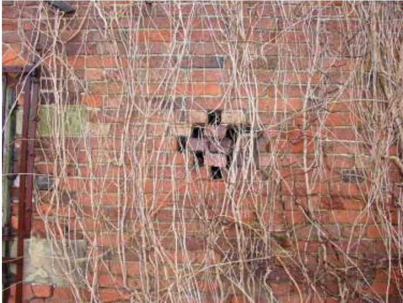
Plate 4 - View showing honey-combed brickwork ventilation
