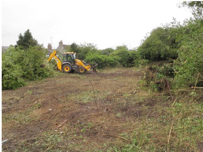
Plate 2 – Clearing site for trenching, looking west from entrance
