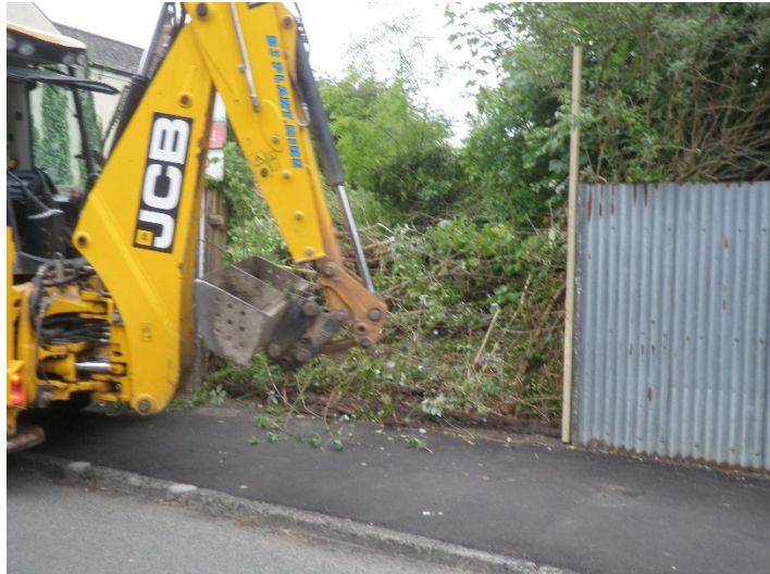
Plate 1 – Site entrance looking southwest, showing overgrowth
