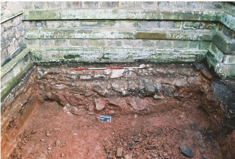
Plate 3 - General view following excavation showing the foundations to the tower, looking south
