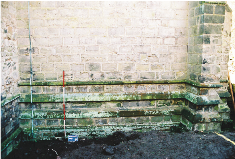
Plate 5 - North facing elevation of the tower, prior to excavation, looking south
