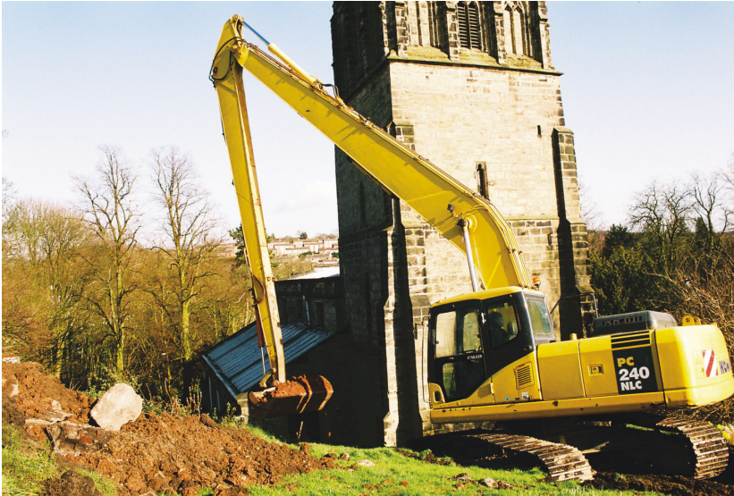
Plate 1 - General view of the development area during excavation, looking southeast
