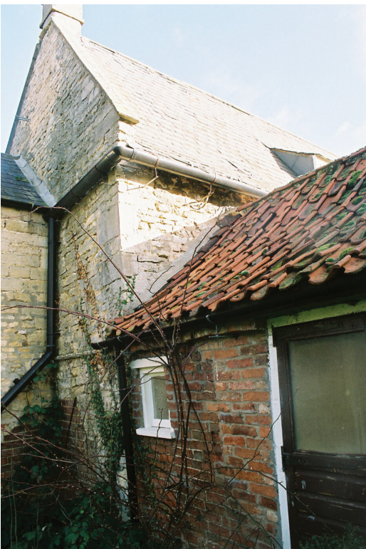
Plate 3 - Detail showing relationship between the extension and principal building, looking northeast
