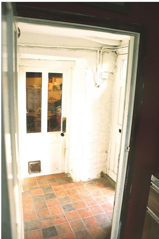
Plate 5 - View showing the lobby area, with door to main cottage in the background, looking north
