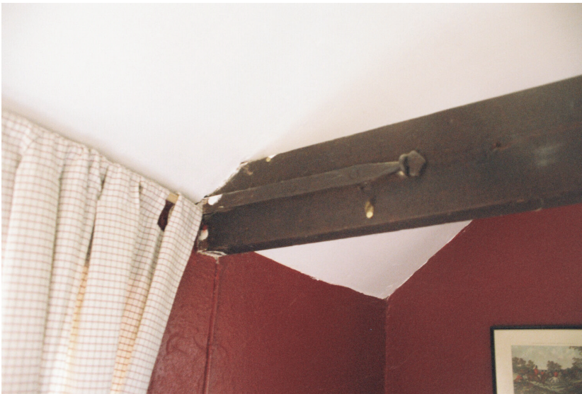
Plate 8 - Detailed view of the tie-beam showing metal clasp
