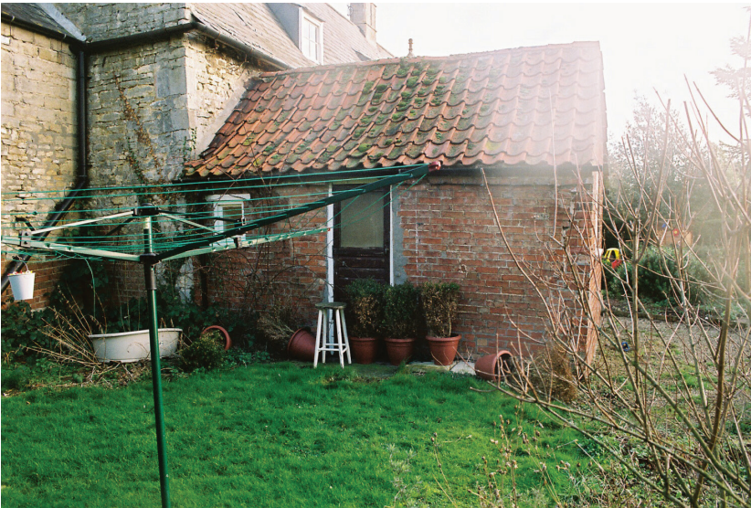
Plate 2 - The west facing elevation showing narrowed doorway, looking east
