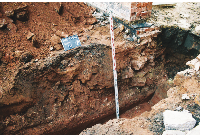
Plate 3 - Section 1 showing the foundations of the extant wall (007), looking south
