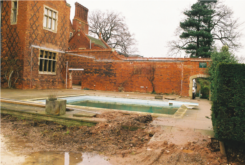
Plate 1 - View looking north across the development area prior to groundworks
