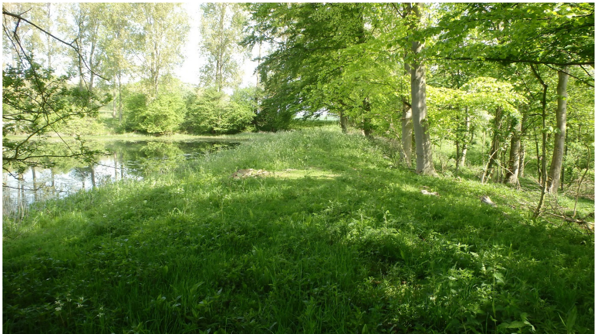
Plate 4 – View along top of dam, looking north
