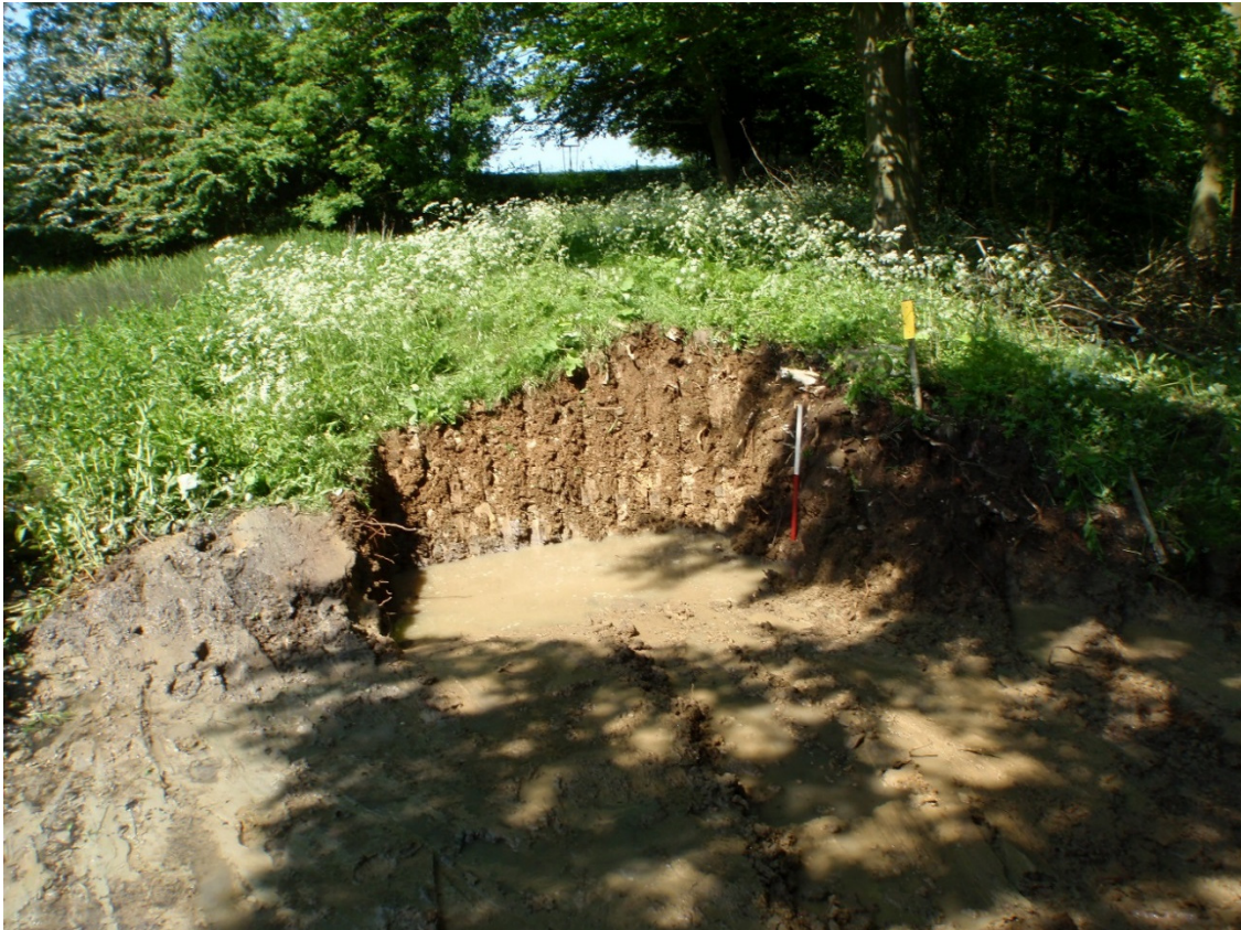
Plate 9 – Excavation of the breach in the dam, Section 1, looking north
