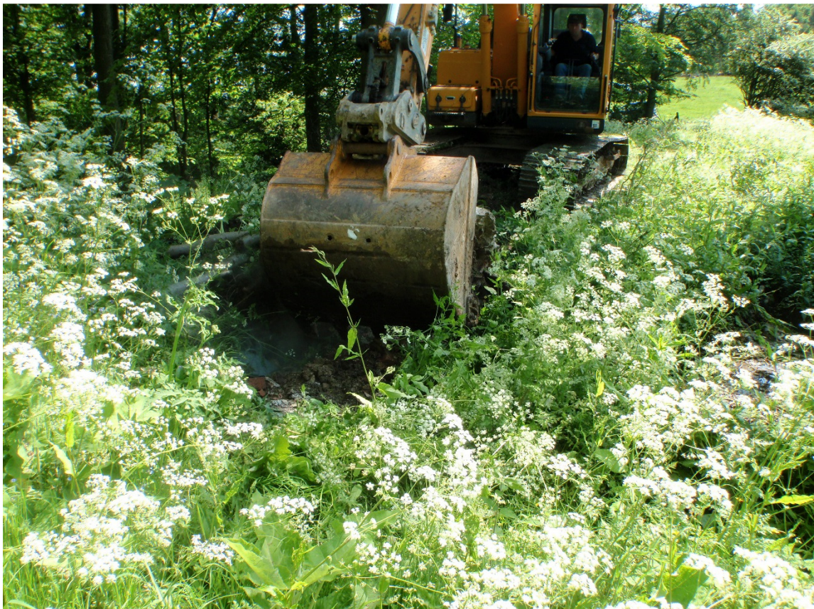
Plate 8 – Excavating the breach in the dam, looking south
