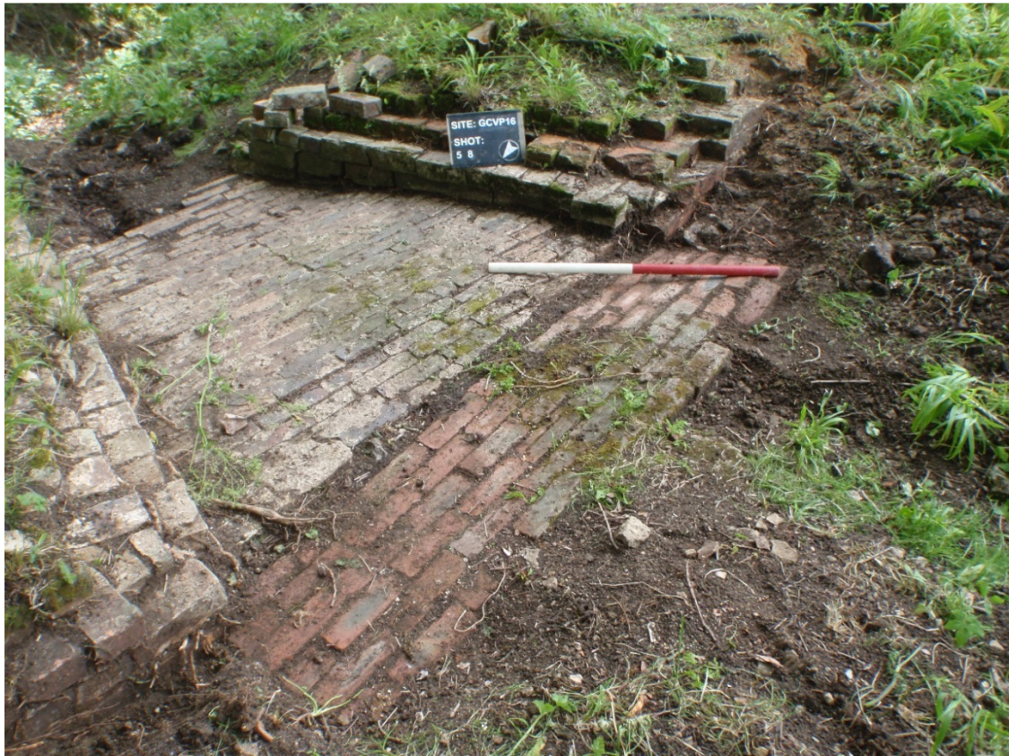
Plate 10 – Spillway entrance, looking southeast
