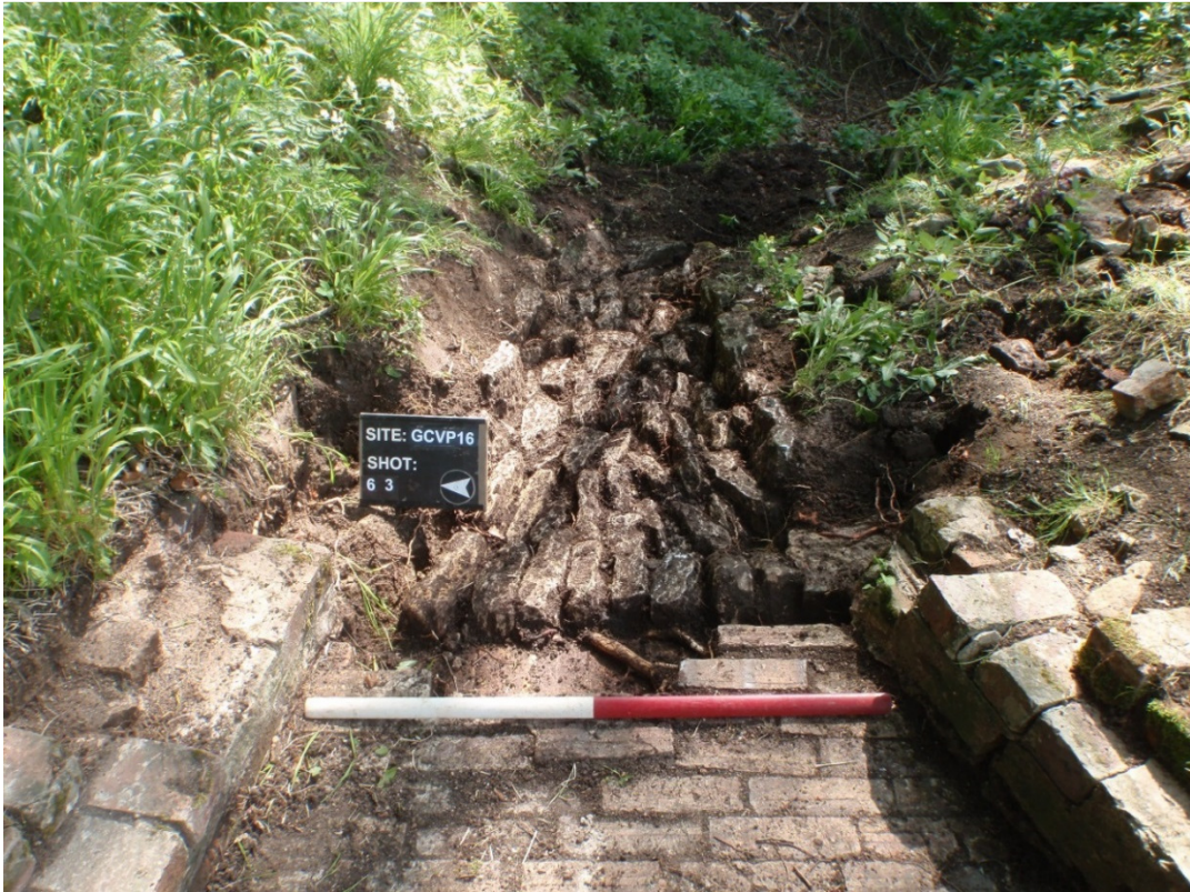
Plate 11 – Eastern end of spillway structure showing stonework (015), (013) and (014)
