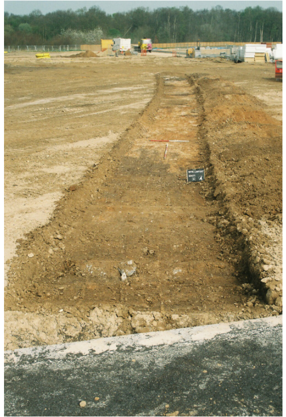
Plate 5 - Trench 4, looking northwest
