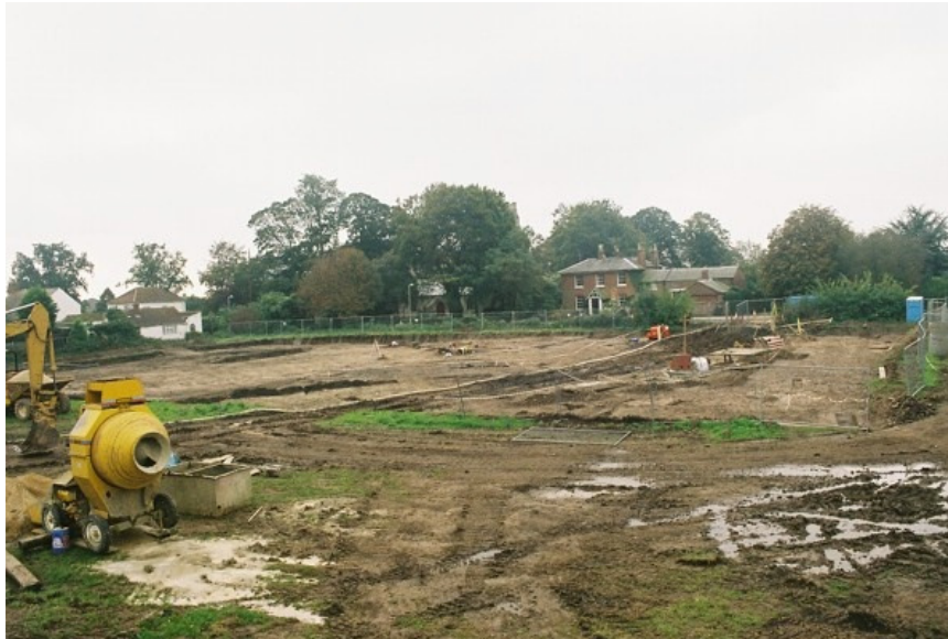
Plate 13 South facing view of site showing construction activity in progress within Area 1
