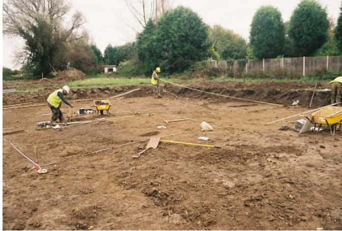
Plate 12 View of northeast corner of site under excavation
