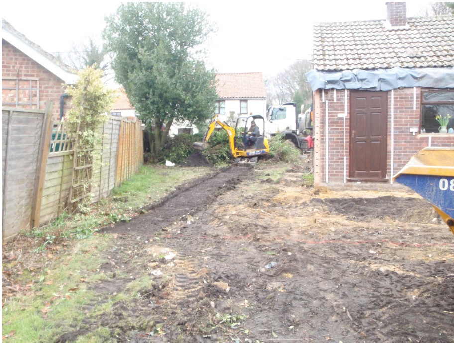
Plate 1. Stripping turf and topsoil, looking north
