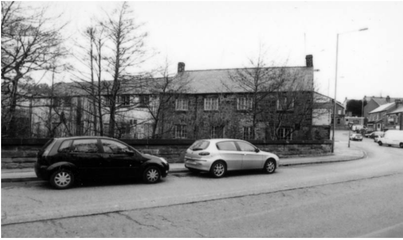
Plate 5 Southern Elevation of E-W Range, looking north
