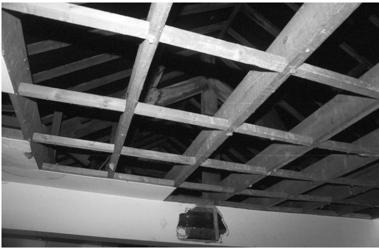
Plate 9 King Post Roof Truss in E-W Range, looking east
