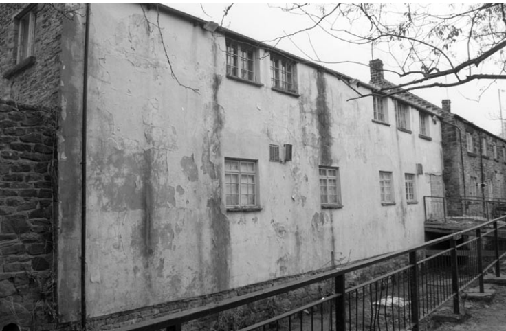
Plate 15 Southern Elevation of E-W Range, showing western end, looking northeast
