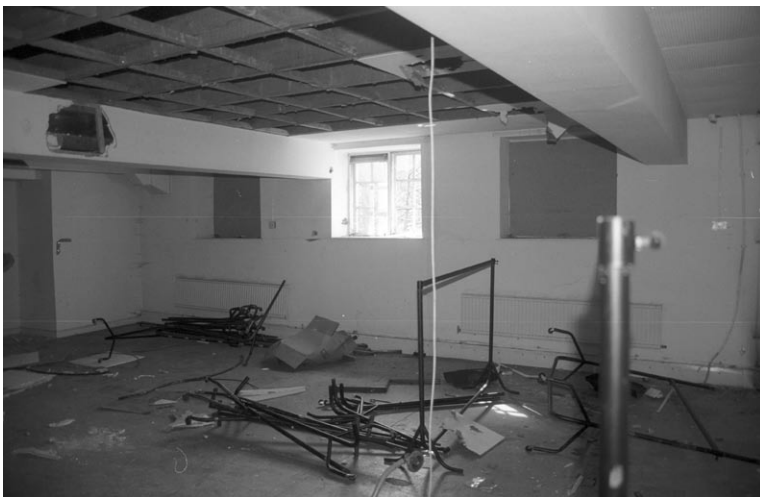
Plate 10 First Floor, West Room of E-W Range, looking southeast
