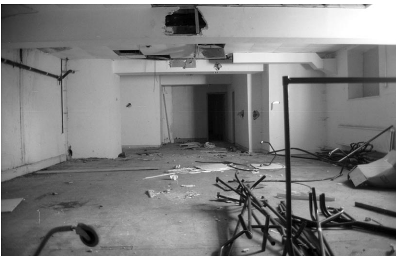
Plate 8 First Floor, West Room of E-W Range, looking east
