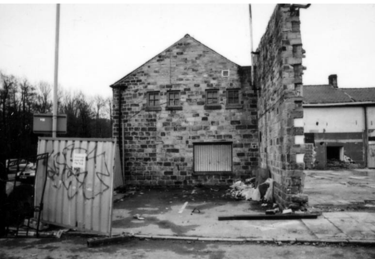
Plate 4 North Gable of N-S Range, looking south
