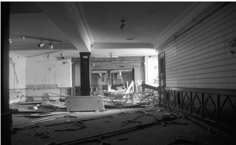
Plate 7 Ground Floor, East Room of E-W Range, looking west
