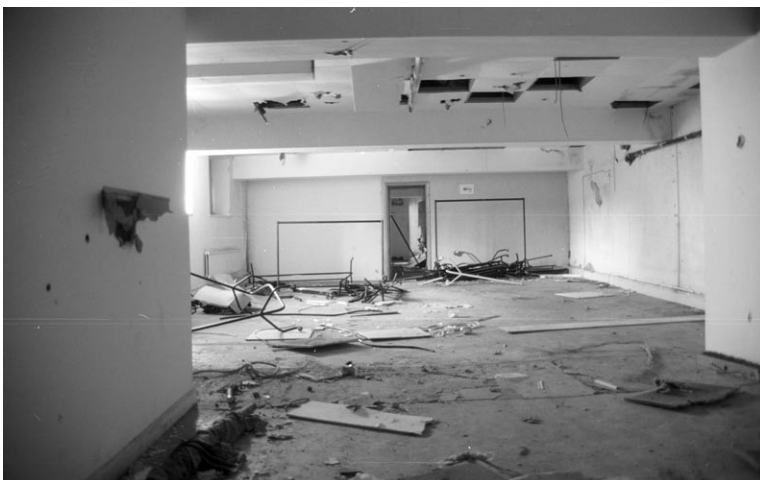
Plate 11 First Floor, East Room of E-W Range, looking west
