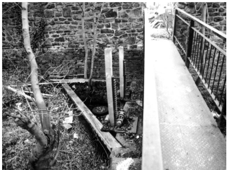
Plate 20 Sluice Gates by southwest corner of mill, looking north
