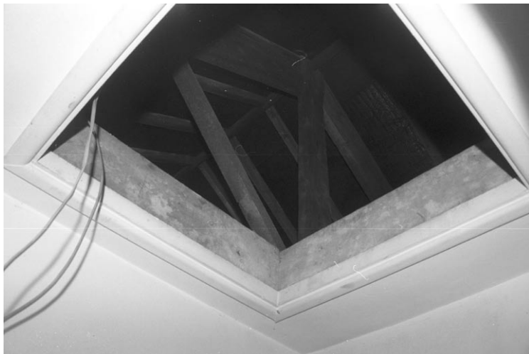
Plate 3 King Post Roof Truss in N-S Range, looking southeast
