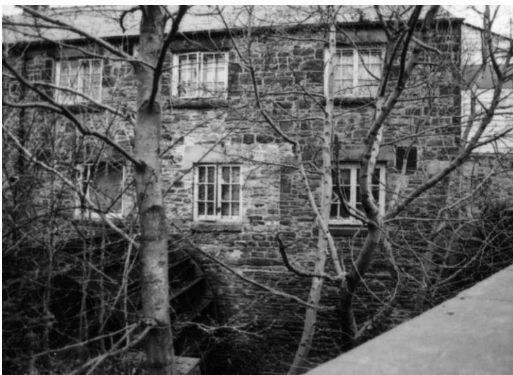
Plate 16 Southern Elevation of E-W Range, showing eastern end and waterwheel, looking north
