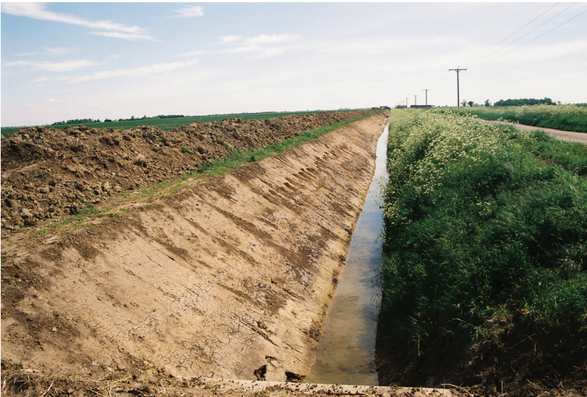
Plate 2 - View of the drainage operations, looking east
