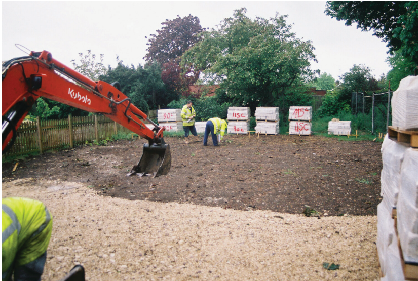
Plate 1 - View looking southeast across the development area
