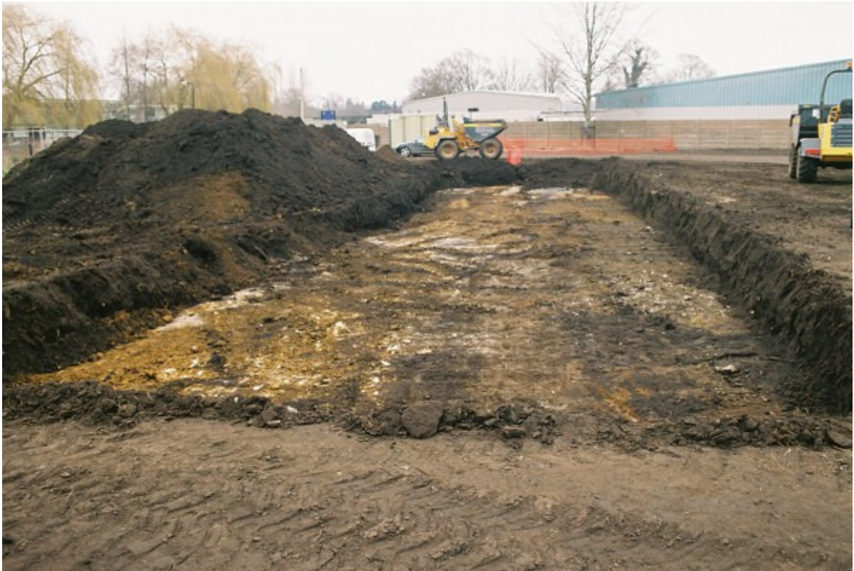
Plate 1 Machine stripping of excavation area viewed from the northeast.
