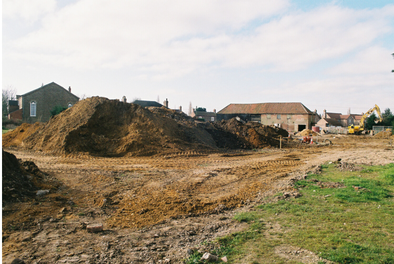
Plate 1 – General view of the Access Road area, looking southwest
