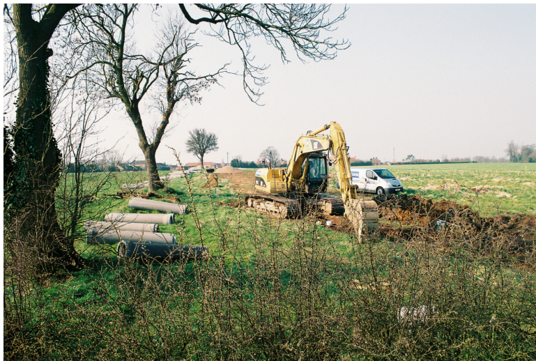
Plate 3 – View looking along the route of the drainage trench, looking southwest
