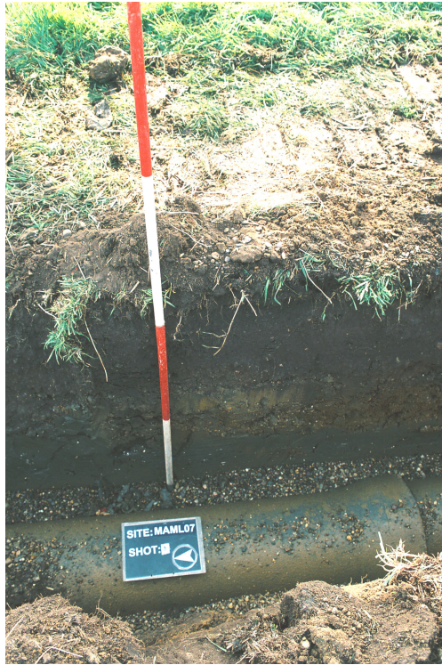
Plate 4 – Section 2, looking southeast
