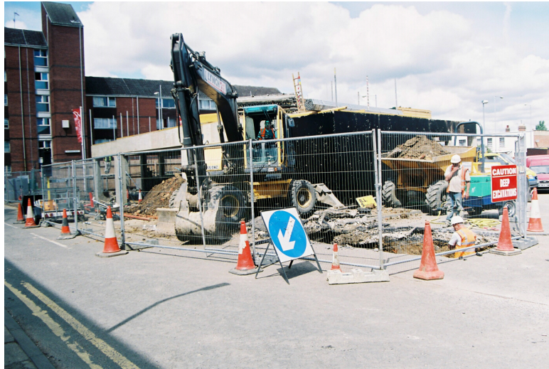
Plate 1 – General view of the development area, looking northwest
