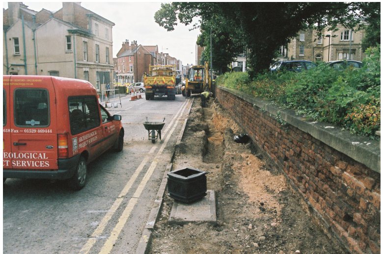
Plate 2 – View of the service trench during excavation, looking west
