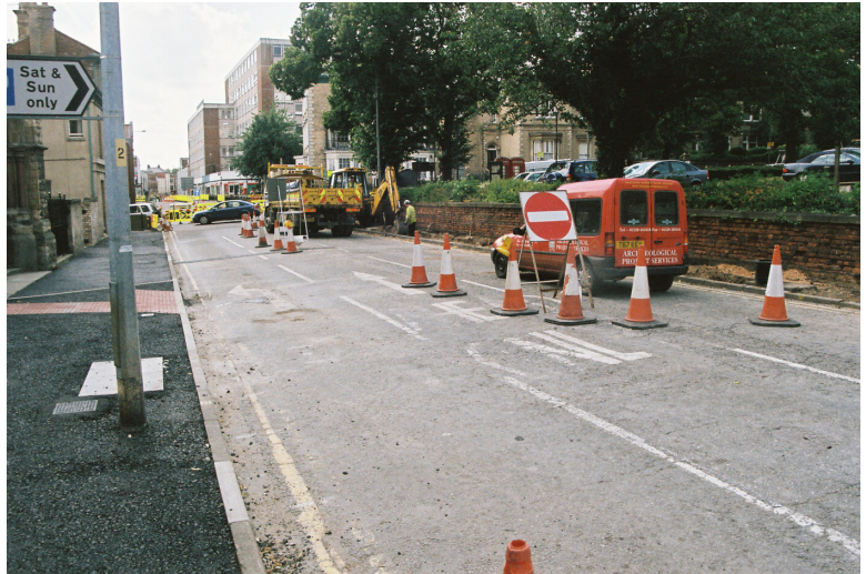
Plate 1 – General view of the groundworks, looking northwest
