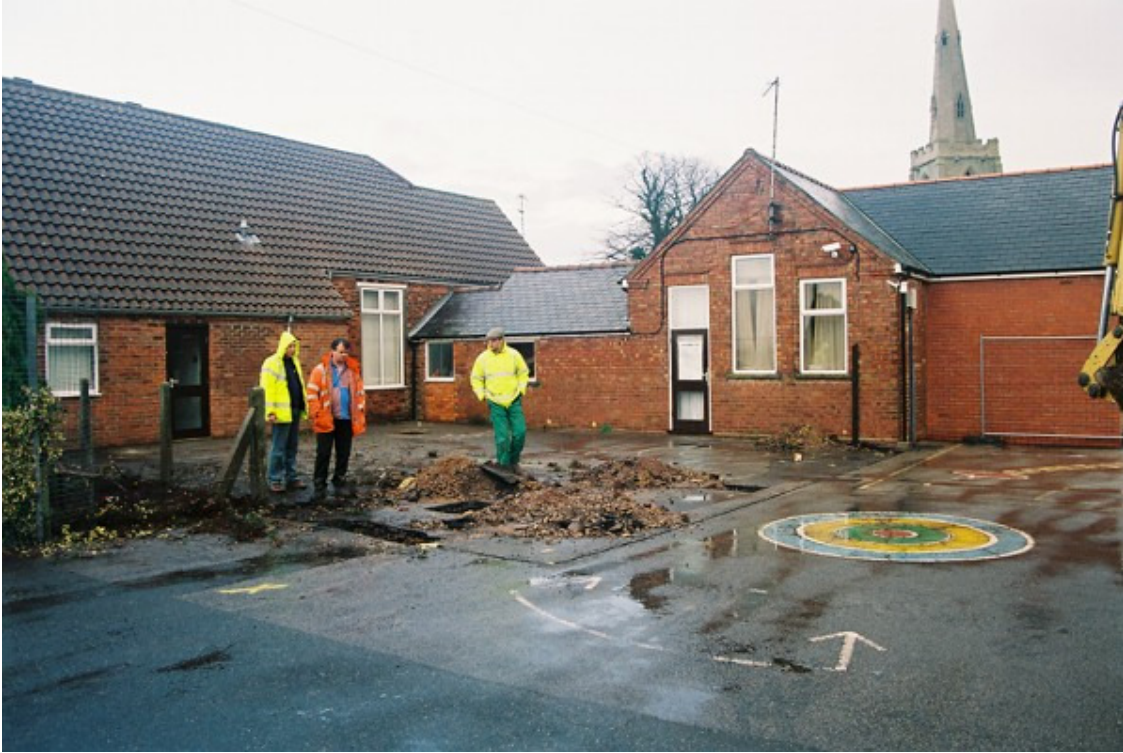
Plate 1: General view of site before removal of tarmac
