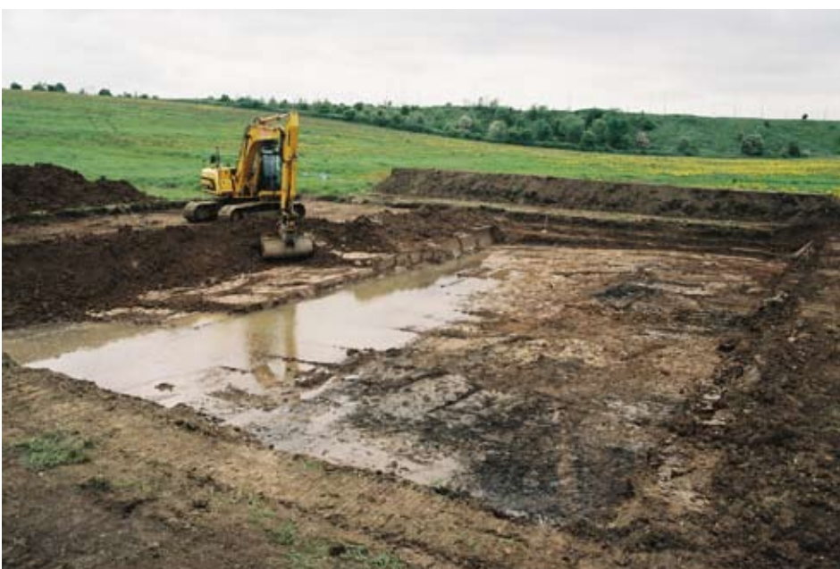
Plate 3 Machining in progress showing occupation horizon (022) in foreground, looking SW
