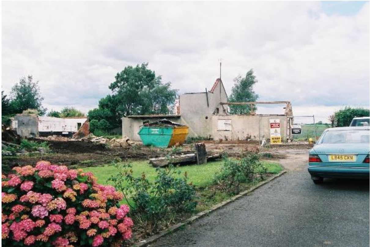
Plate 1. General view looking northwest during demolition
