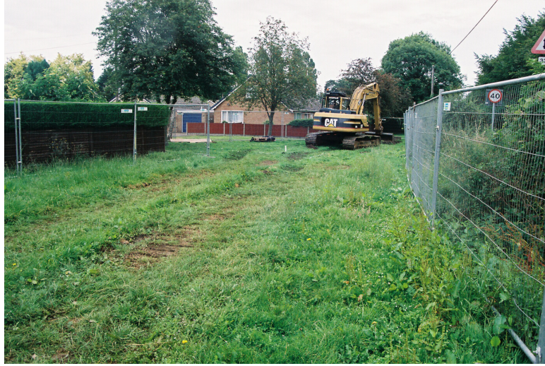
Plate 1 – General view of the development area, looking east
