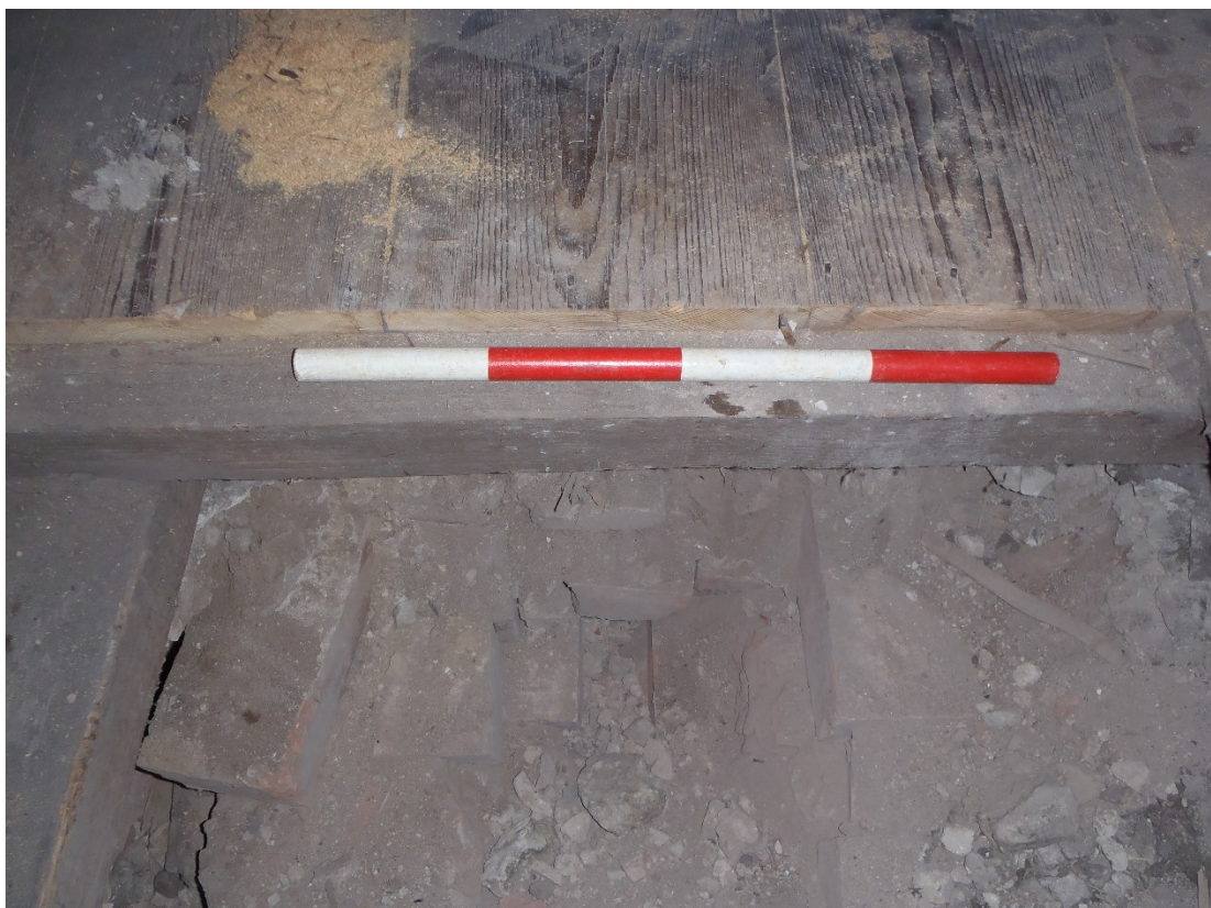
Plate 4 - Trial pit 2, abandoned due to solid brickwork, looking east
