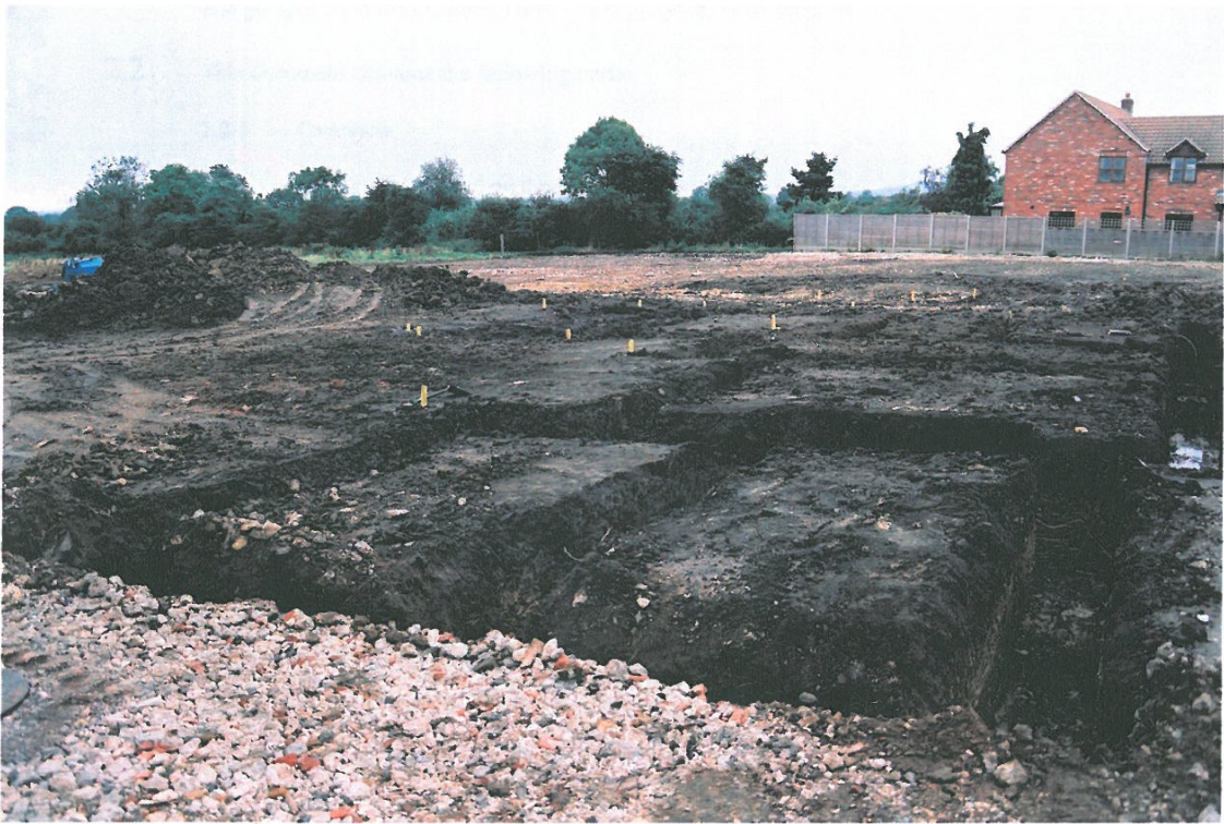
Plate 4. Completed footings looking northeast
