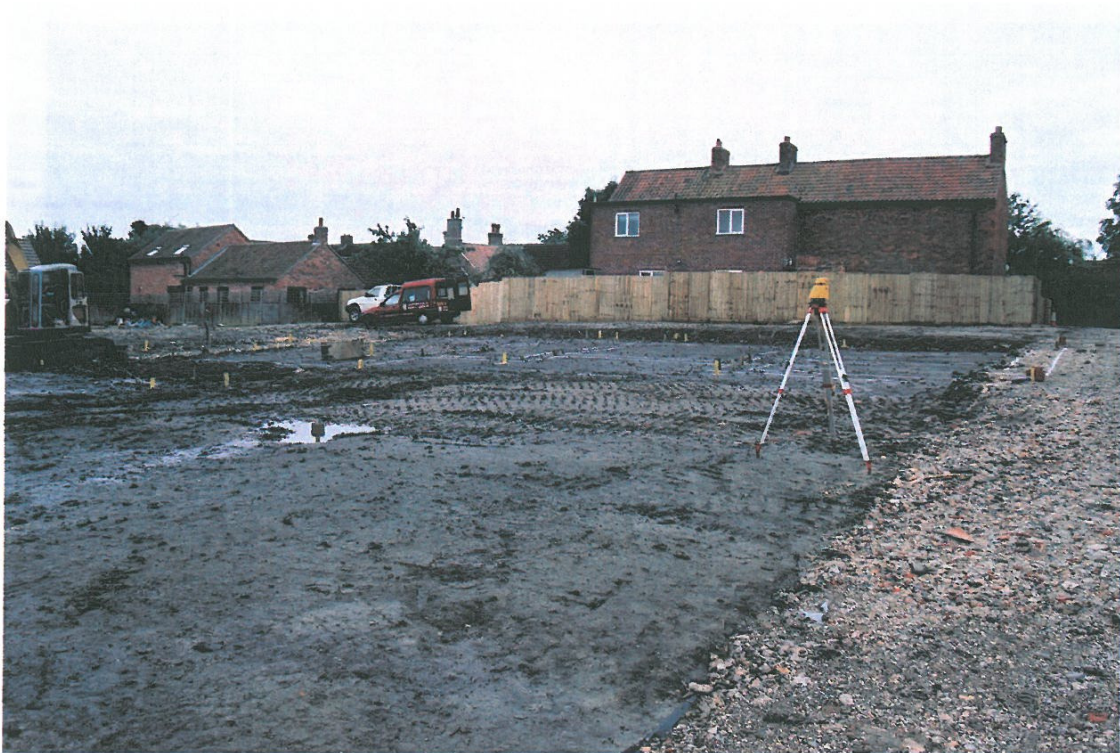
Plate 1: Pre-excavation view looking SE towards farmhouse
