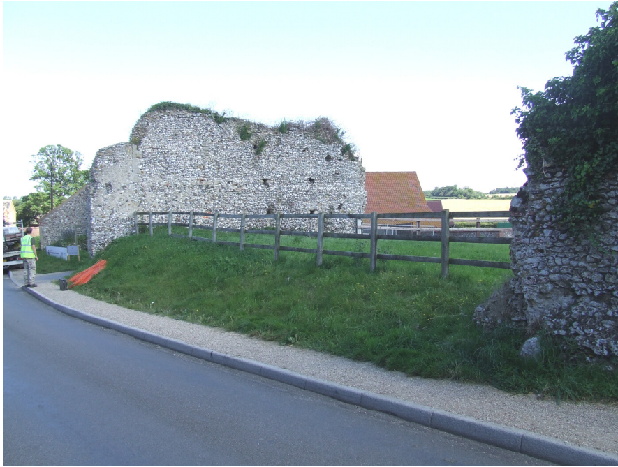
Plate 1 – View of the area under investigation, looking north
