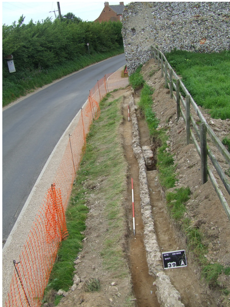
Plate 2 – The exposed medieval precinct wall (218), looking northwest
