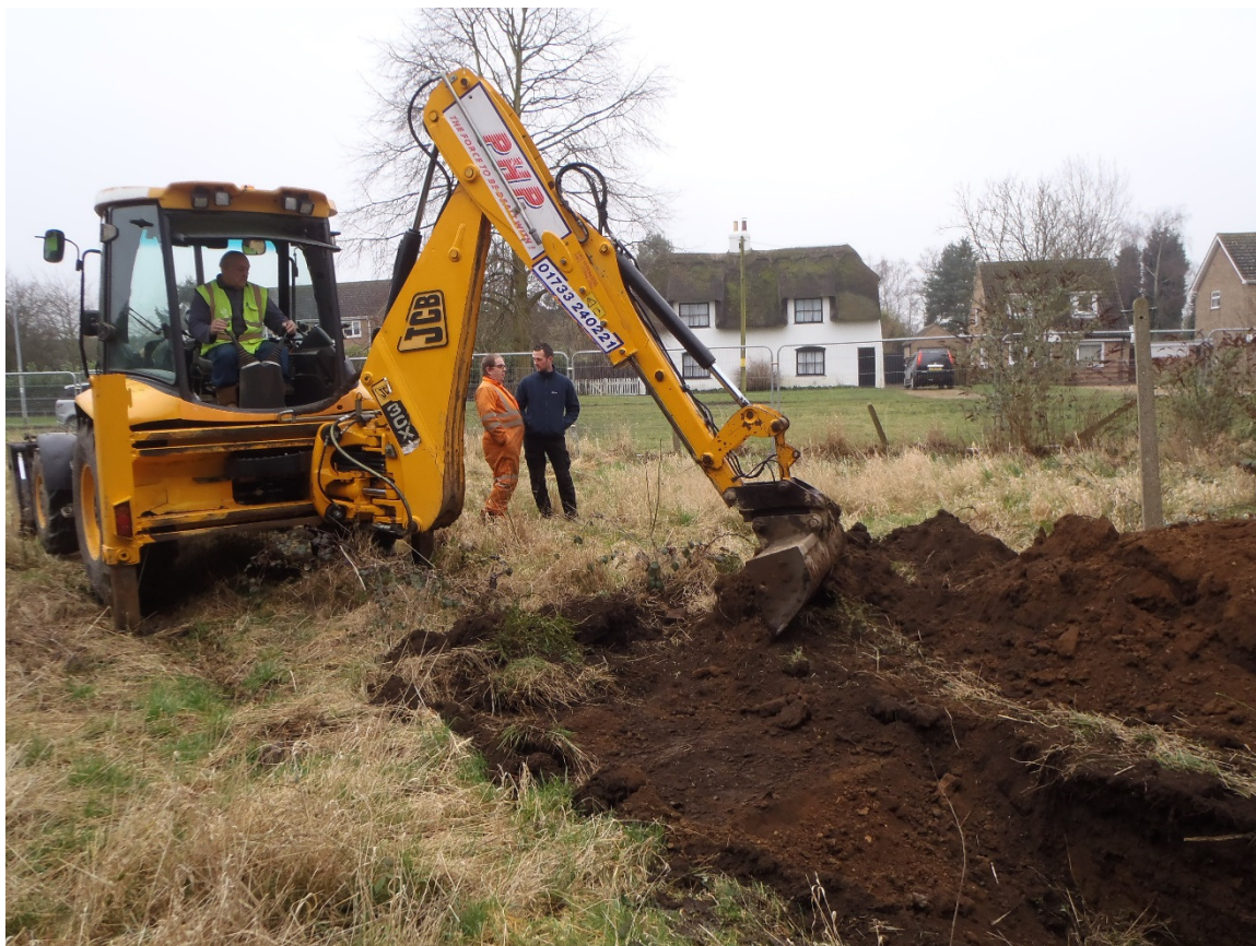
Plate 4 Machine digging Trench 1.
