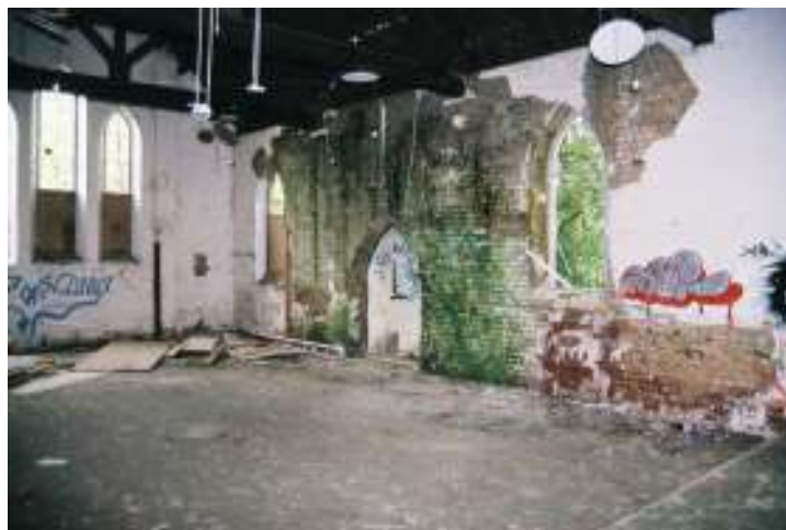
Plate 3 – Interior view of the chapel, looking northwest
