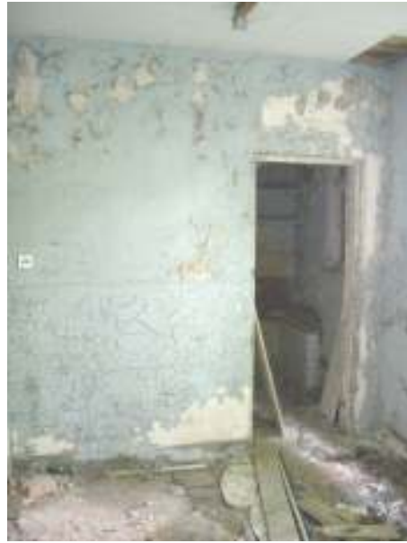
Plate 10 – Rooms B and D, looking west
