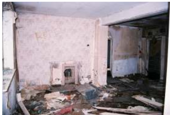
Plate 12 – Room E, looking north
