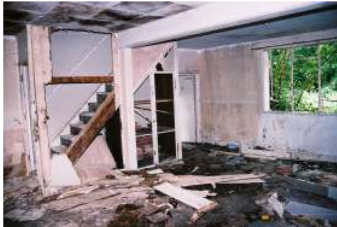
Plate 11 – Room E, looking south
