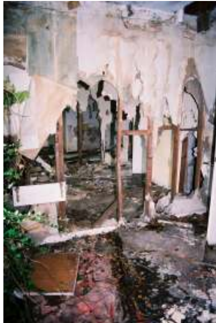
Plate 14 – View of the first floor, looking southwest
