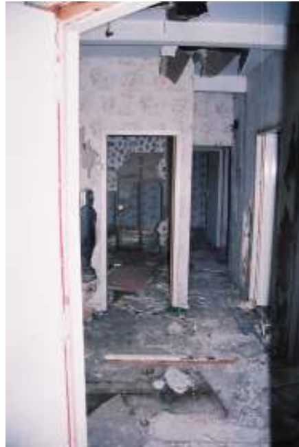
Plate 13 – View of the first floor, looking north from the stairwell
