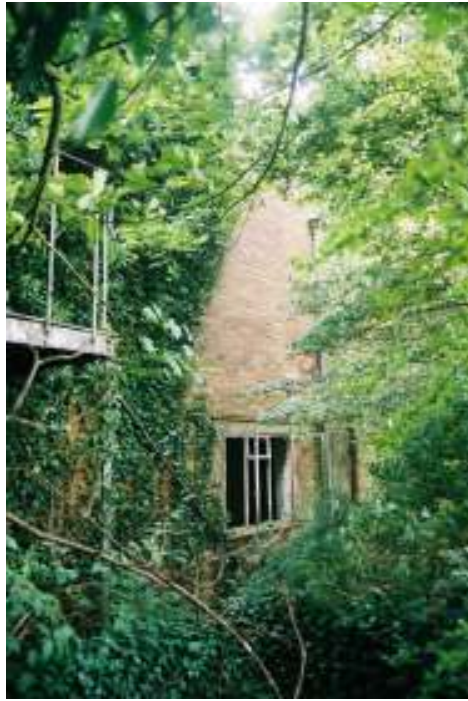
Plate 7 – The north façade of Rowan House
