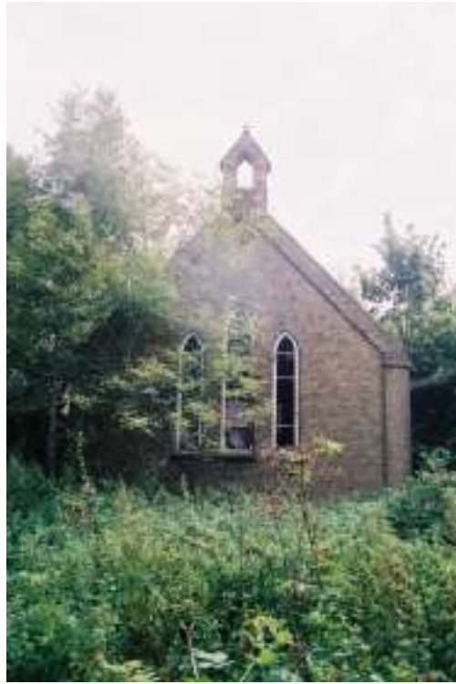
Plate 1 – View showing the west façade of St Lawrence's Chapel
