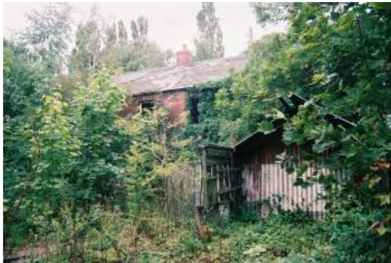
Plate 5 – The east façade of Rowan House
