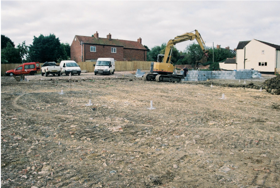
Plate 1: General view of Plot 2 machining looking towards old farm house
