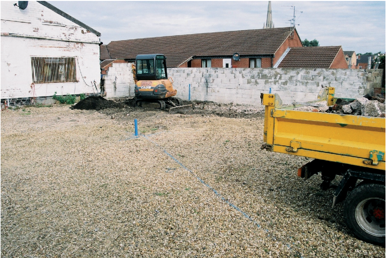
Plate 2 General view of site, looking NW
